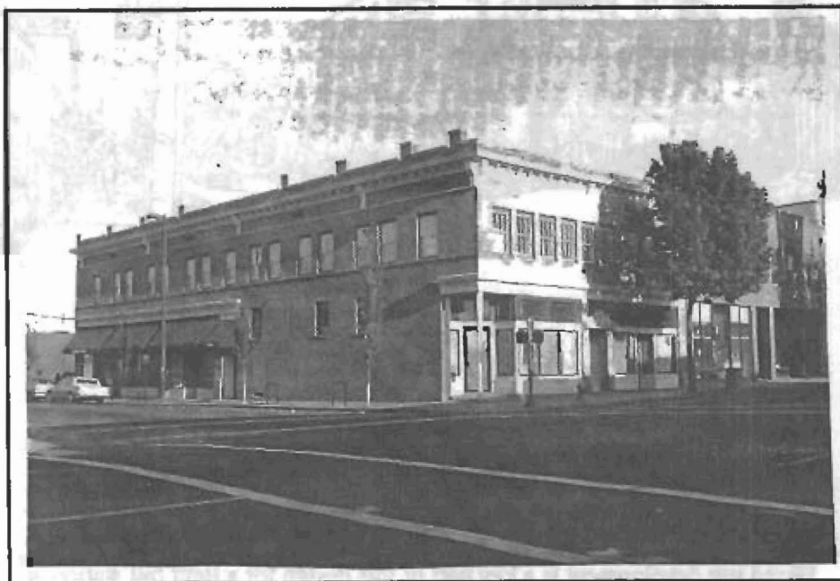
The Smart Building on Martin Luther King Jr. Blvd. was recently rehabilitated. Doris' Cafe is one of the new tenants.
