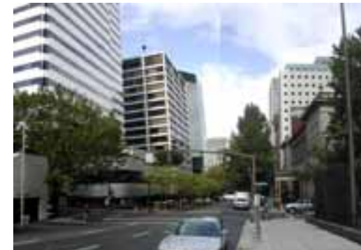
Future platform location at City Hall/PacWest
