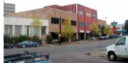
SW 5 th Ave. looking south from College
