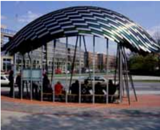
Uniquely designed and more sculptural light rail shelters would contrast with the staid facades of nearby buildings and can enhance the vibrancy of the adjacent plaza (source: Big Ideas, Small Buildings , by Phyllis Richardson)
