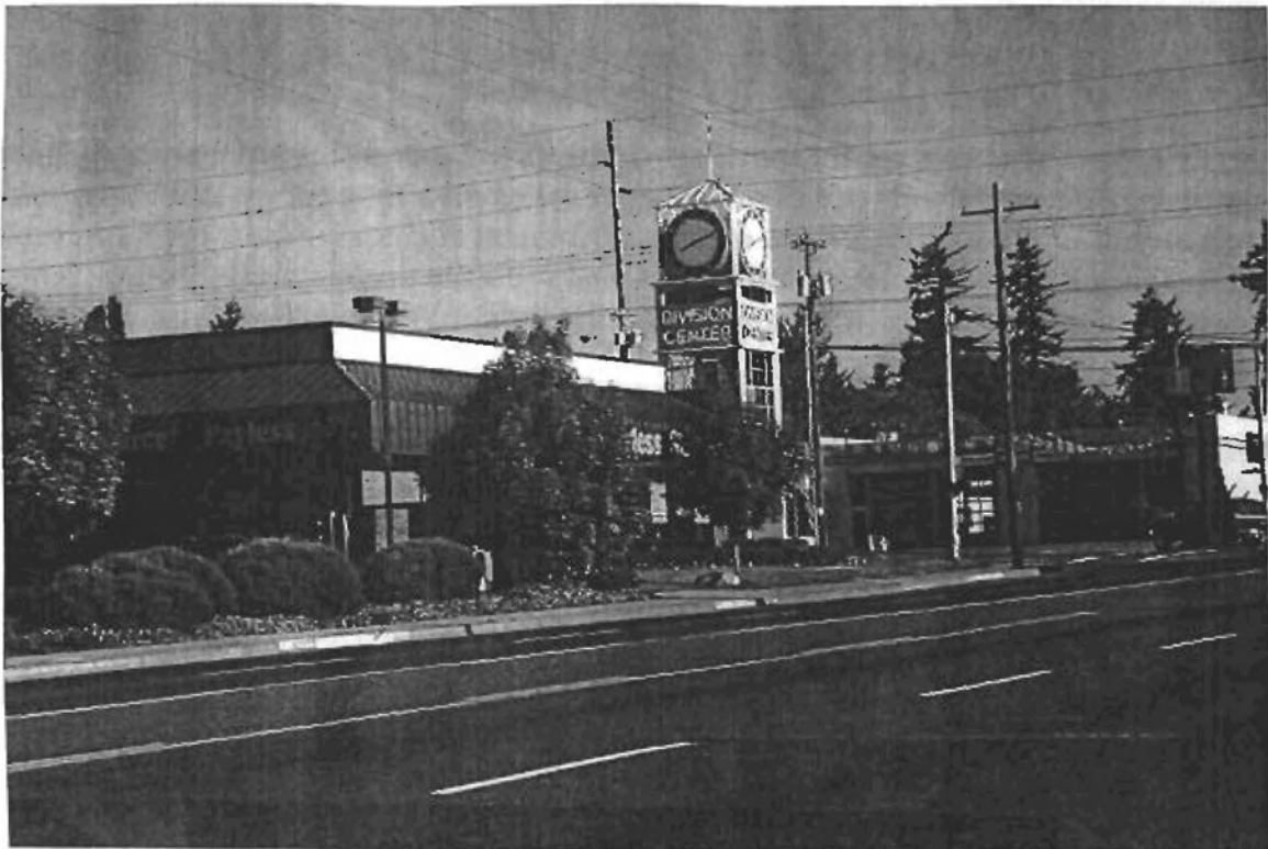
Division Center at 122nd and Division
