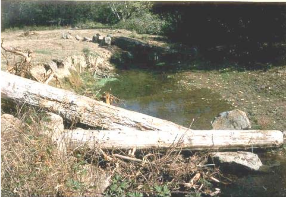
Photo 4. 1993 photo taken just after structure placement in North Fork Indian (Mann Creek) Note raw eroding banks and lack of woody vegetation.
