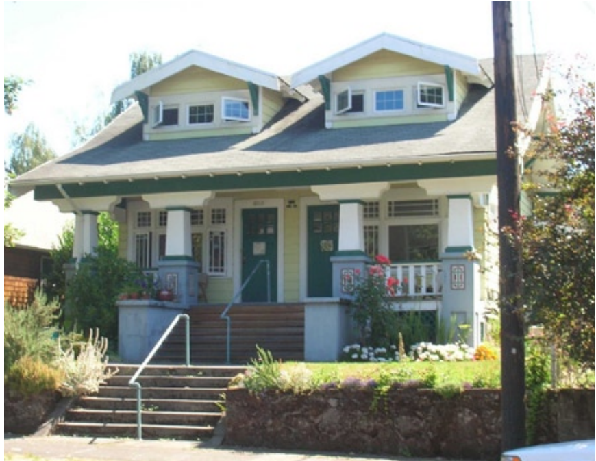
Duplex bungalow (1907) with upper-level living space within dormers, an arrangement common in the early 20th-century bungalows that predominate in many Portland neighborhoods.
