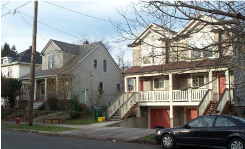
Rowhouses with excavated lower-level garages
