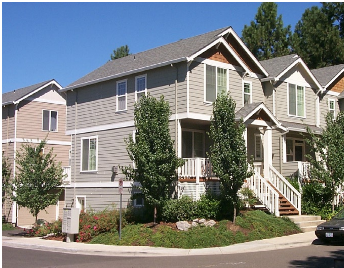
The lower-level, rear accessed garages of these rowhouses are partially-excavated below grade, allowing the upper living space to relate strongly to the street (providing a street relationship similar to historic patterns of houses built over partially-excavated basements).
