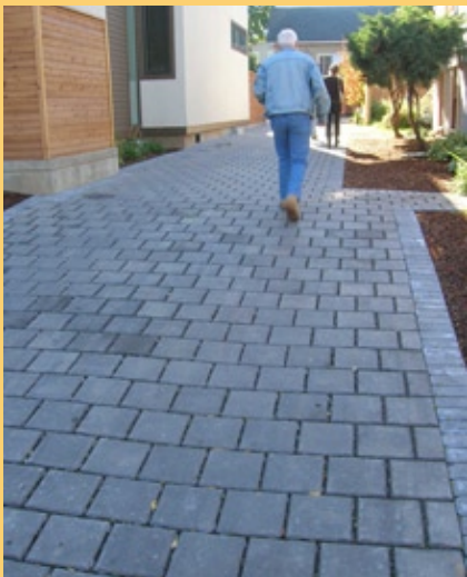
Driveway (above), surfaced with paving blocks, providing shared pedestrian and vehicle access to rear buildings and parking—a space-efficient alternative to requirements for grade-separated walkways (top).
