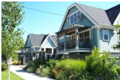
The single vehicle accessway of this six-unit shared court project minimizes disruptions to the neighborhood streetscape, while street-fronting units continue patterns established by nearby early 20th-century houses (Eastern Crossing, Seattle)
