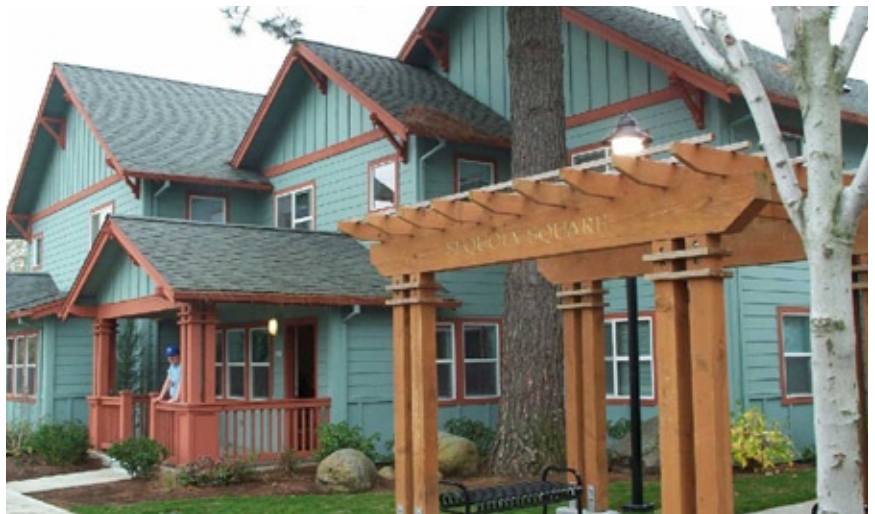
Apartment project in Outer East Portland, with façade divided into "house-like" building volumes.
