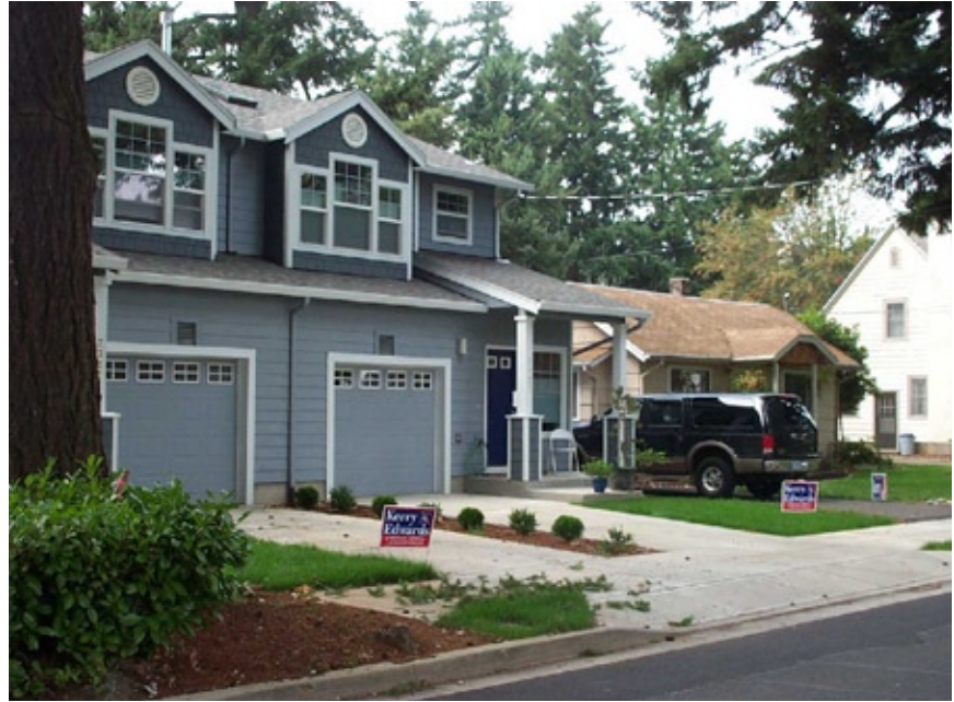
Roof forms set at single-level height help mitigate the scale contrast between these paired rowhouses and the adjacent small cottage.
