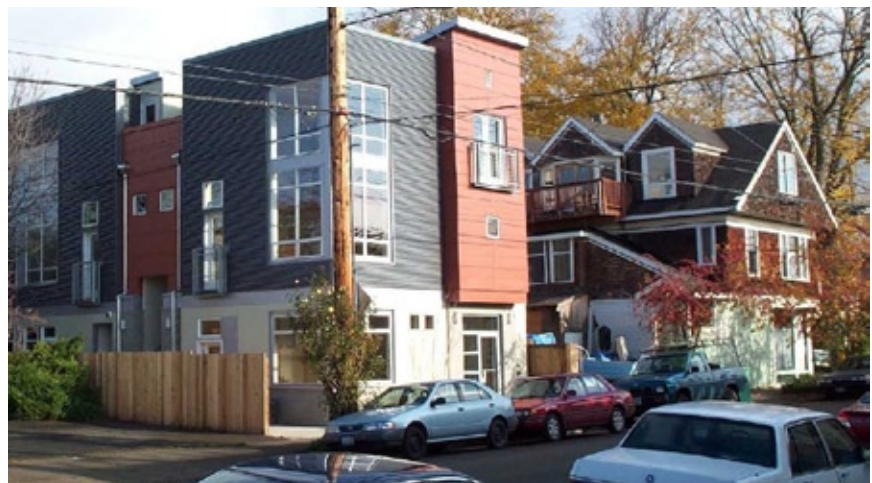
7-unit structure (built 2004) with no off-street parking on a 4,000 sq.ft. site. Includes 4 townhouse condominium units (over 3 ground-level studio units), which sold quickly. Developer related that buyers were more concerned about adequate bicycle storage than the lack of off-street parking.
