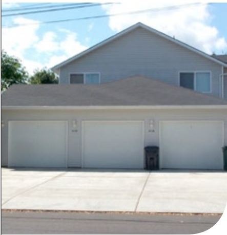
Integrating parking in ways that do not dominate the site is one of the greatest challenges of designing infill projects
