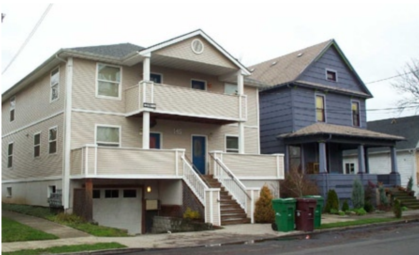
Fourplex with excavated basement parking
