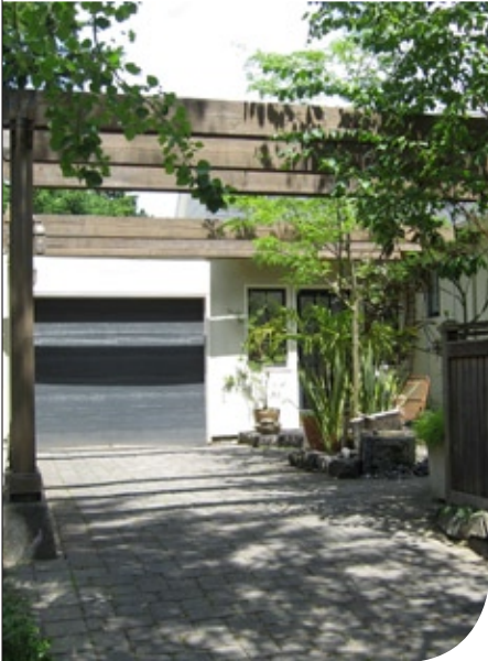
Driveway designed as extension of patio space
