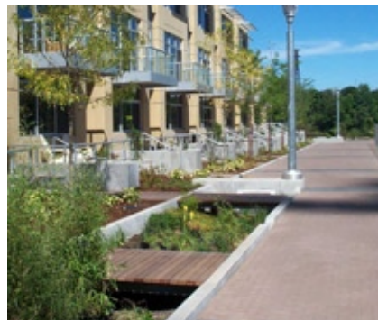
Stormwater planters integrated into the design of shared pedestrian/vehicle space (Meriwether Townhouses)
