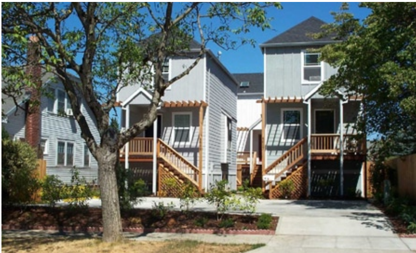
Cluster of detached houses with excavated basement living space
