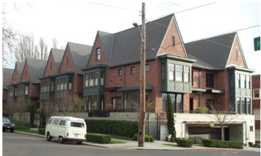
Townhouses (Victoria Townhomes, Seattle—1999), basement parking shared with adjacent building
