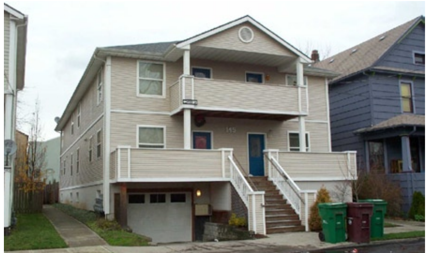
Fourplex (1997) with basement parking (see case study, page XX).
