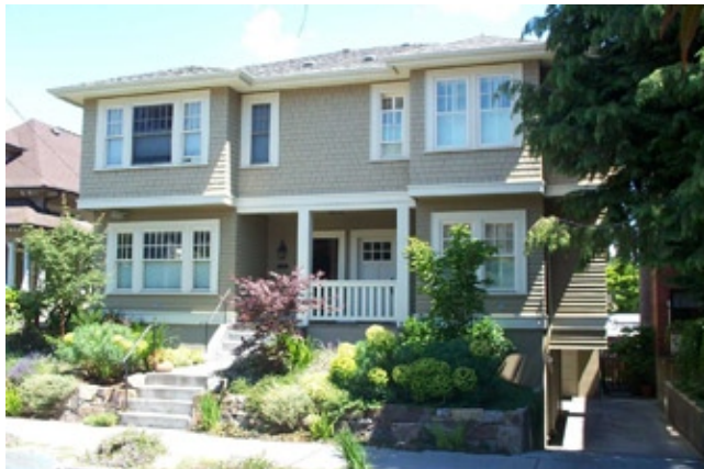
Four-unit townhouse cluster in Seattle, with partially-excavated garages.
