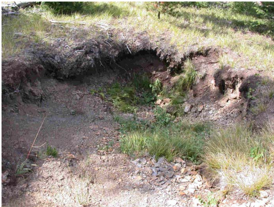
Photo 10. Large depression above Adit #2. (Photo by D. Boles)
