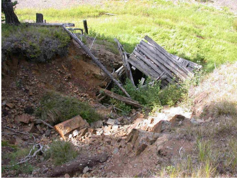
Photo 9. Partially collapsed adit at Portal #2. (Photo by D. Boles)
