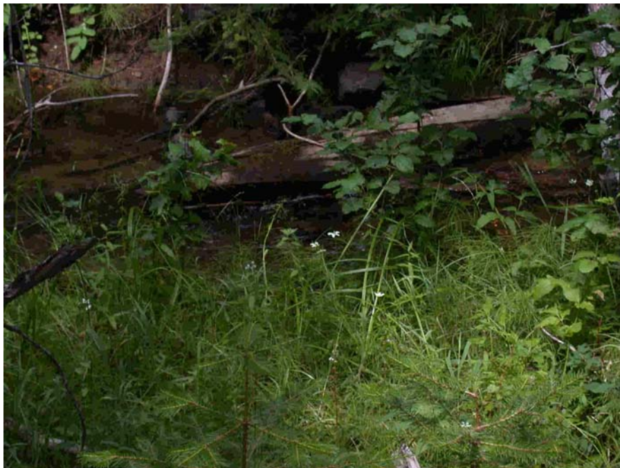
Photo 12. Collapsed Adit #3. Lat/Long: 44° 50' 42.8"N/118° 24' 08.8"W (Photo by D. Boles)
