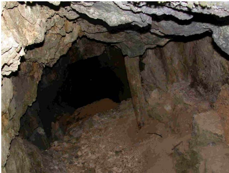
Photo 18. Inside view of Adit #5 shown in Photo 17. (Photo by D. Boles)
