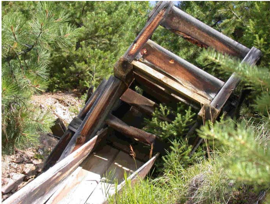
Photo 4. Close-up of hopper. (Photo by D. Boles)
