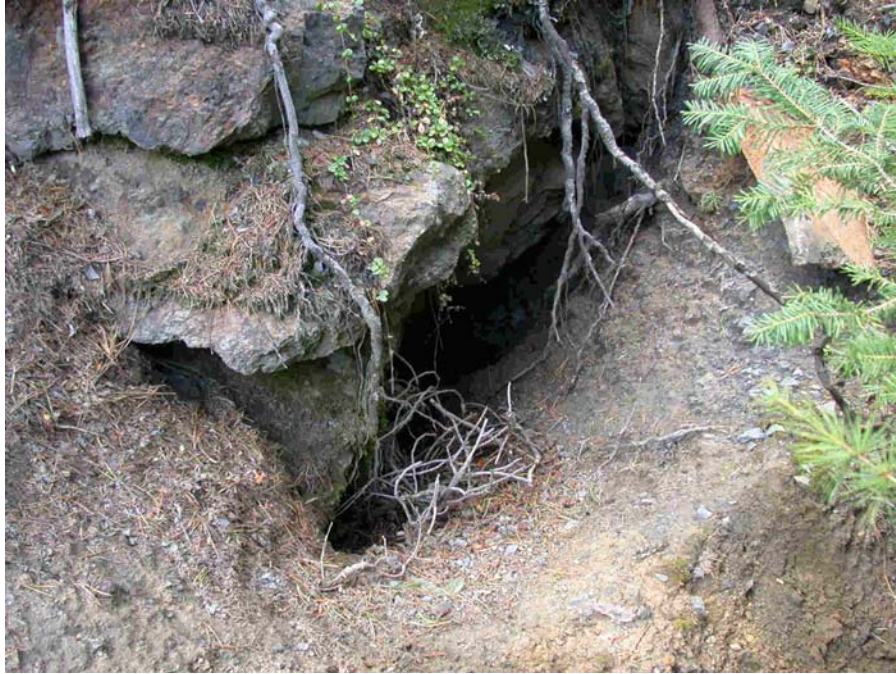
Photo 11. Partially collapsed New York Adit #4. Lat/Long: 44° 50' 43.3"N/118° 24' 10.1"W (Photo by D. Boles)
