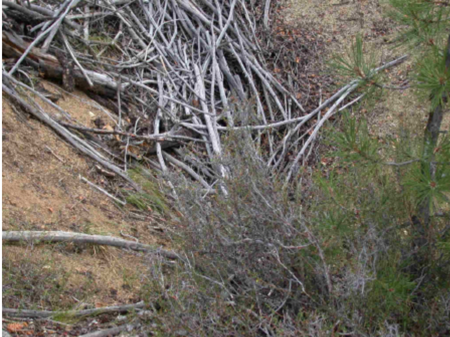
Photo 1. Secondary collapsed adit. (Photo by D. Boles)
