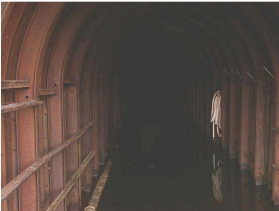
Photo 2. Inside Portal at the 600 Level (Photo by D. Boles)
