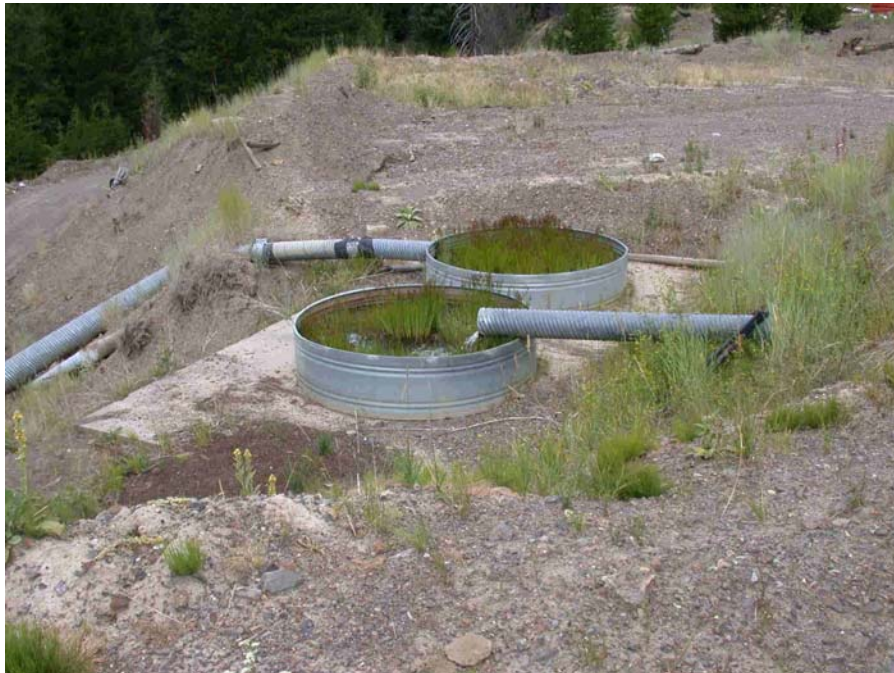
Photo 6. Discharge tanks below treatment pond #2. (Photo by D. Boles)
