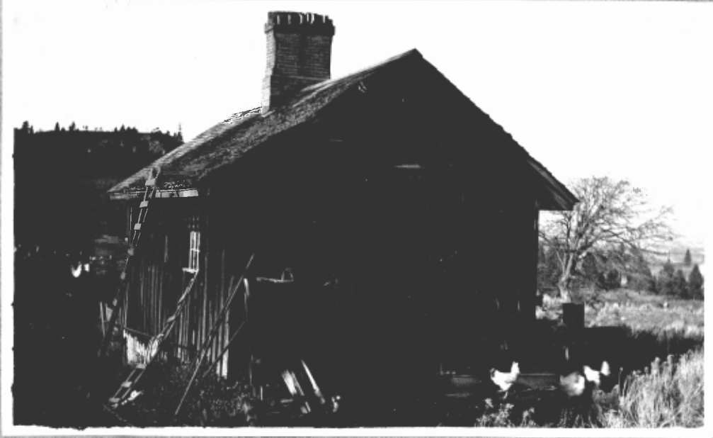
The bakery for the fort which is still occupied by the old baker.
