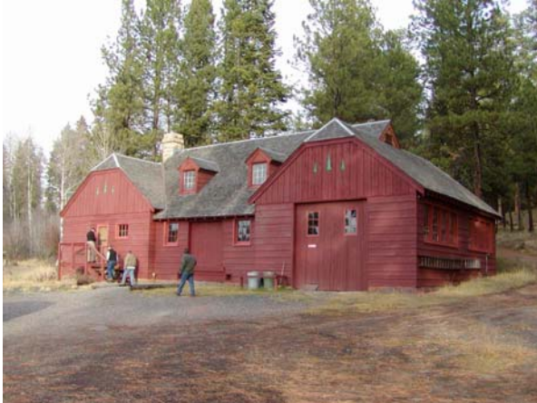
Photo 2: Existing Allison warehouse/bunkhouse
