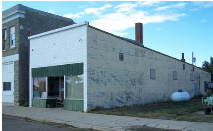
MT Lumber and Hardware Building, 2007, photo Laura Nowlin
