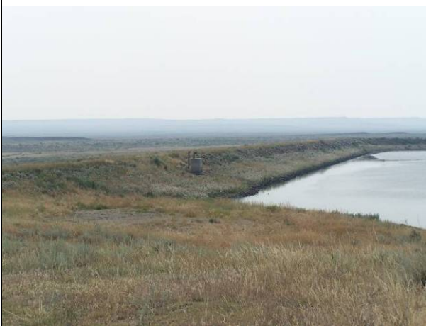
Northwest side of Yellow Water Dam, 2007, photo Laura Nowlin
