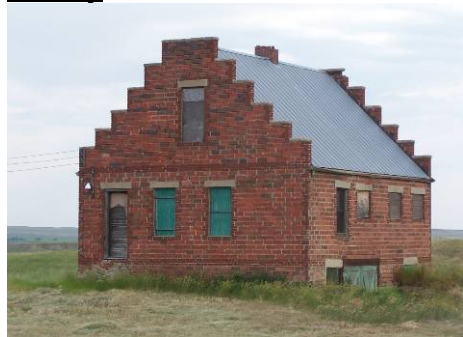
Old Brick House, 2007, photo Laura Nowlin
