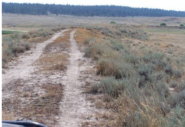
West end diversion dam, 2007, photo Laura Nowlin
