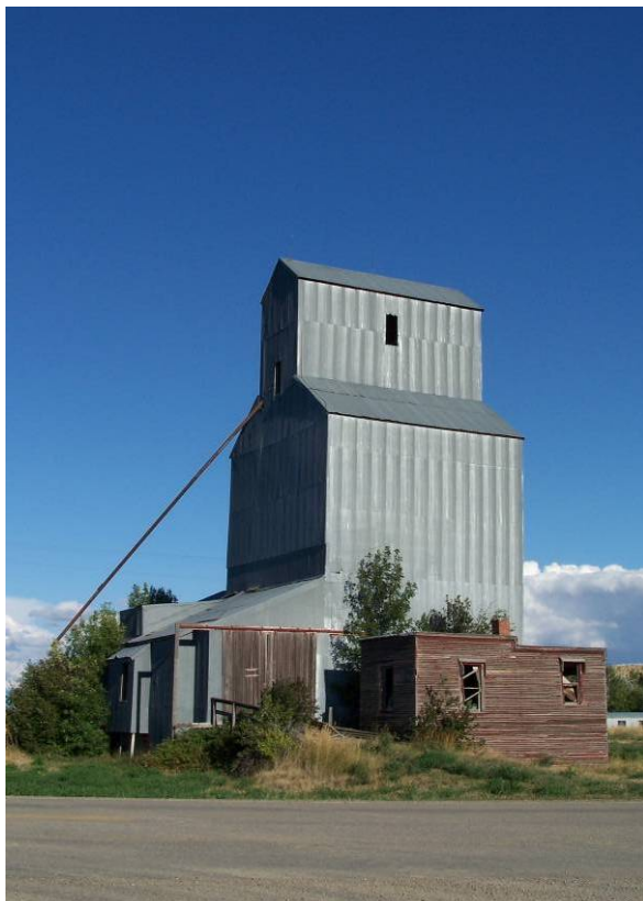
Montana Elevator, 2007, photo Laura Nowlin
