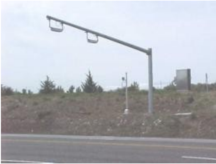
Figure 9. Weigh-in-Motion Overhead Detector
