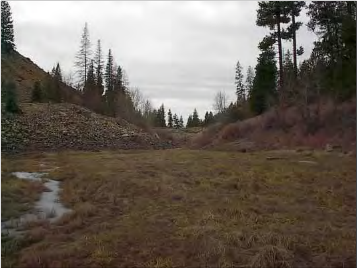
Plate 5-6.6. Canyon Meadows Reservoir, looking downstream at the dam (photograph taken November 19, 2002).
