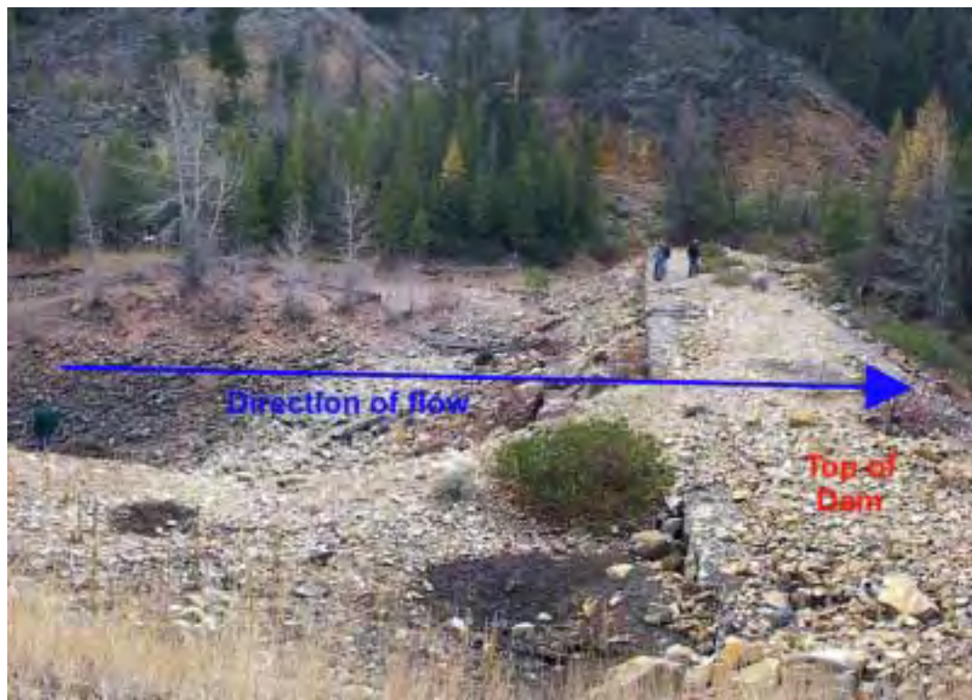
Figure 1.14. Canyon Meadows Dam. Looking south across dam crest. Reservoir pool is located to the left. Photo taken 11/19/2002.
