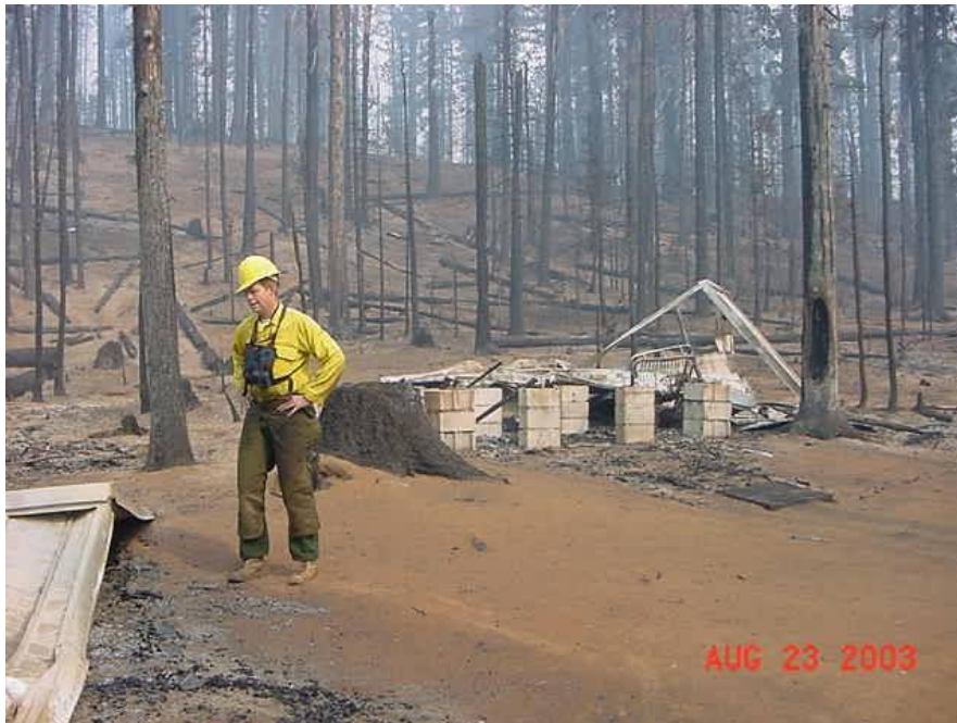
Paul Engstrom surveys Round Lake Christian Camp after the B&B Fire, several structures and vehicles were destroyed
