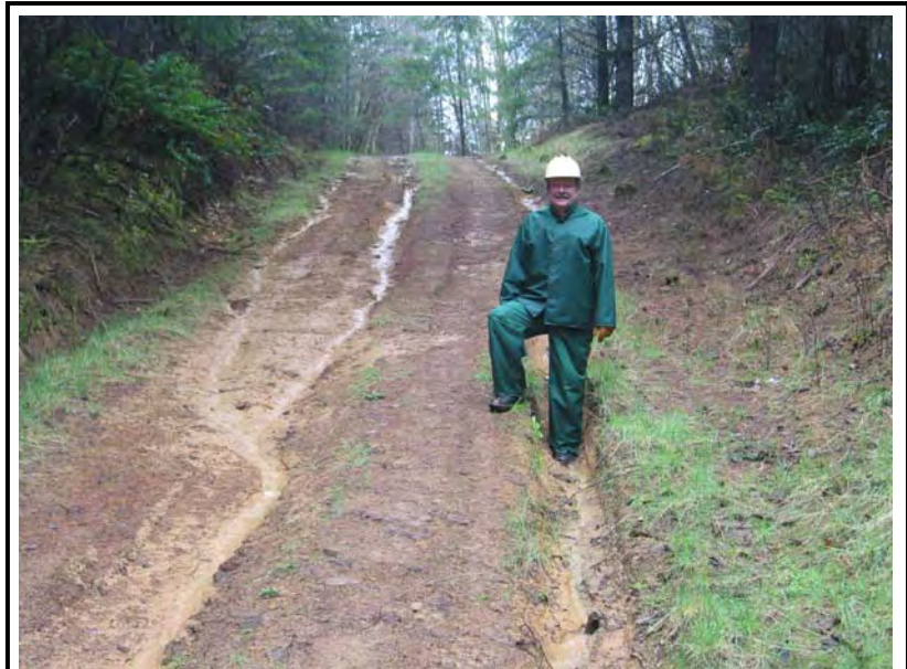
Figure III-5: Erosion on the 22-8-32 road in the Lutsinger Creek-Sawyer Rapids subwatershed. This spur would be renovated for access, and decommissioned following project completion.
