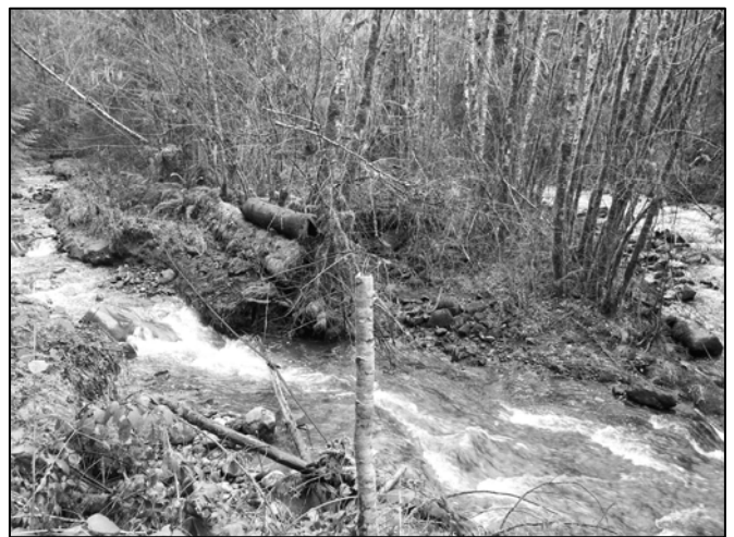
Figure 2. Old road functioning as seasonal channel.
