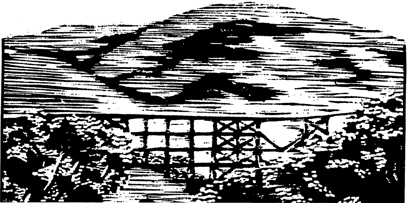
Old railroad trestle at Gordon Canyon
