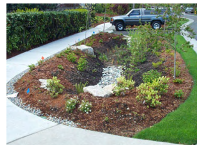
Prototypical “Green Street” improvements in Seattle as part of the SEA Streets program.
