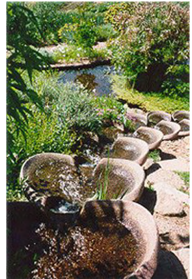
Sculptural flow forms aerate stormwater and improve water quality.
