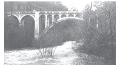
Concrete bridge on Pacific Highway, Oswego Creek, built in 1920 (Janet Banks Collection).
