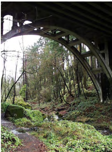
View of Highway 43 Bridge from Oswego Creek ravine.
