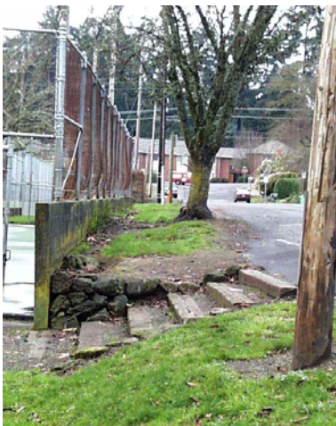
Stairs at Ladd Street into Children’s Play Area.
