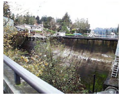
Lake Oswego dam and surge tank.
