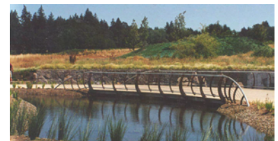
Pedestrian bridge over water quality swale.
