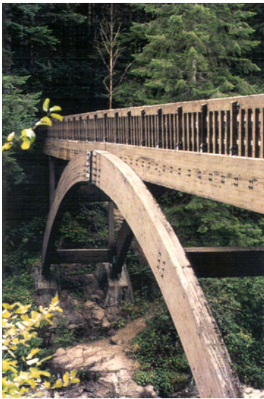
Bridgewalk over Oswego Creek.
