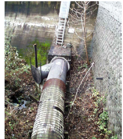
Penstock outlet at dam.
