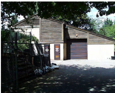
Restroom Maintenance Building - lower level
