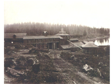
Casting building (left), Furnace (center), and Blast-House (right) at mouth of Sucker Creek, 1867, Carlton Watkins photo (Nickel 1999:127).
