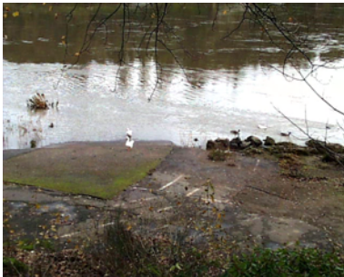
Boat launch in disrepair on Willamette River.
