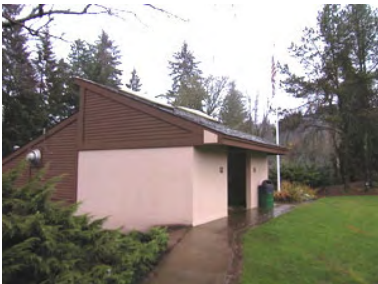
Restroom Maintenance Building - upper level
