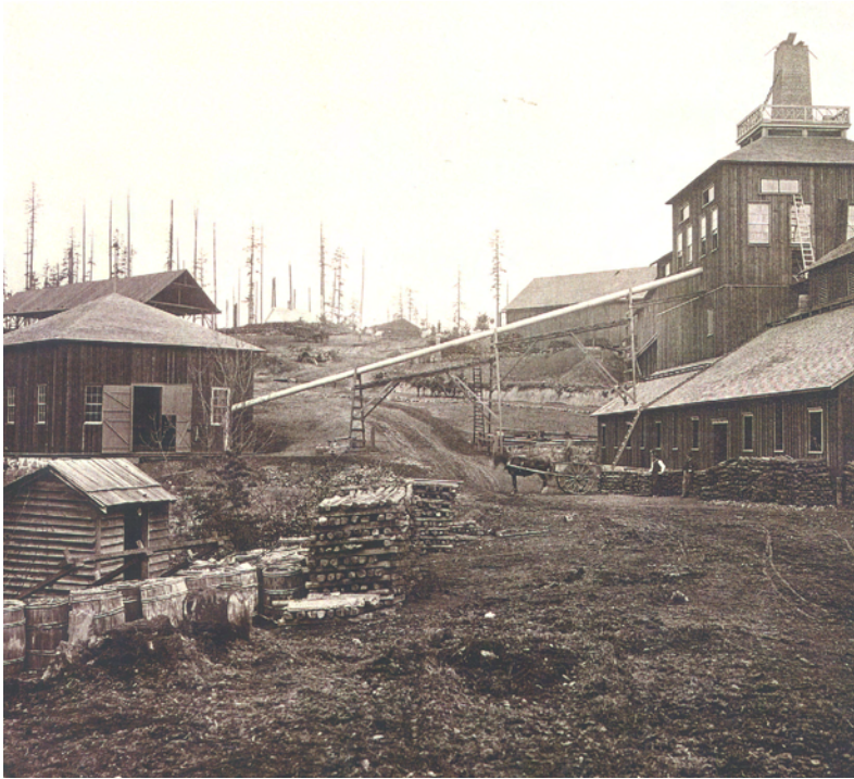
Blast-House (left) and Furnace (right) with stacks of wood for making charcoal, Carleton Watkins, photo, 1867 (Nickel 1999:131).
