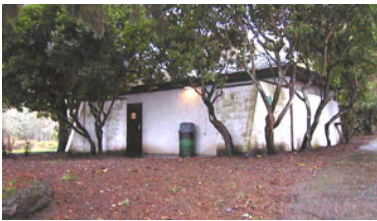
Lower Restroom Building
