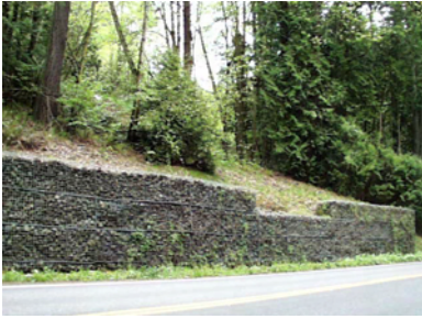
Gabion walls are proposed to support the Green Street parking area in the Oswego Natural Area.
