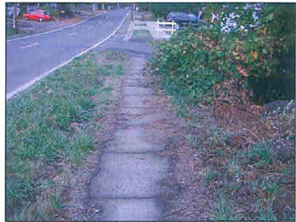
Overgrown shrubs greatly reduce the usable walking surface of many sidewalks, making them inaccessible to many users.
