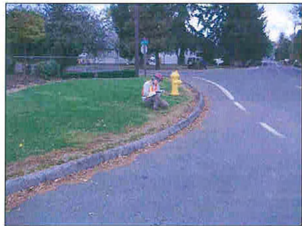
Wynooski is lacking pedestrian facilities west of 11 th Street.
