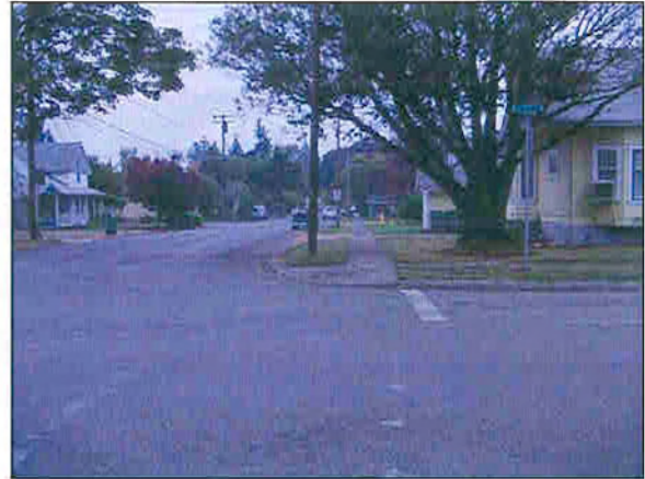
Missing curb cuts south of downtown make pedestrian travel difficult.
