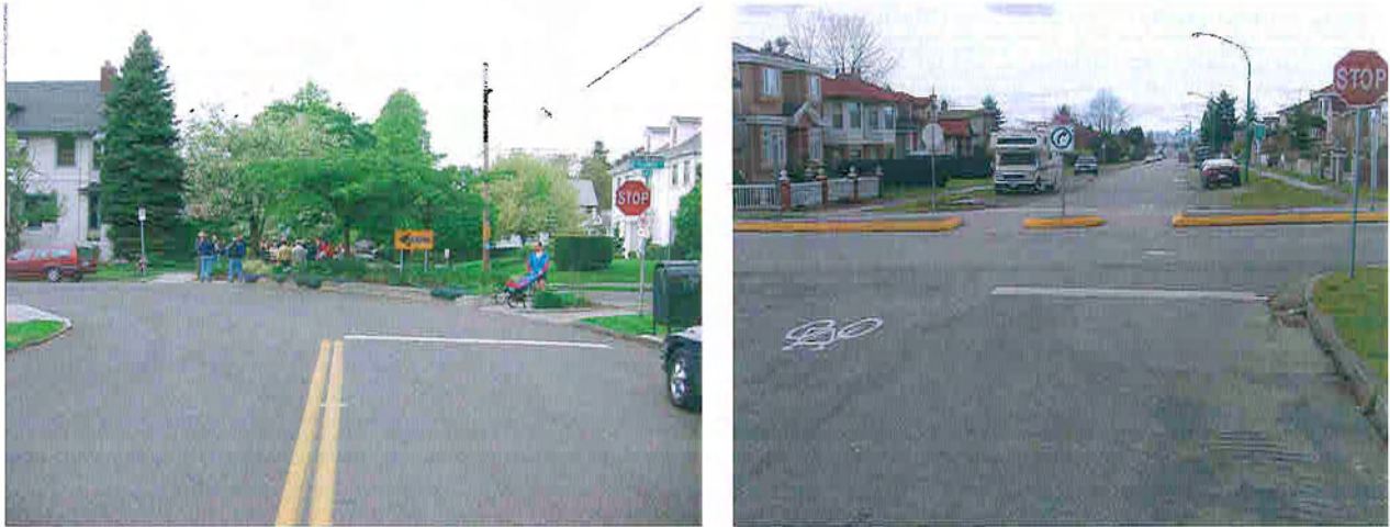
Traffic Diverters: Median island (left) and bike/ped only refuge on NE 16th and Tillamook in Portland, Oregon.
