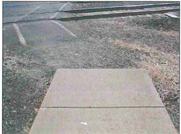
Adding smoother transitions and warning devices will improve pedestrian safety at railroad crossings.
