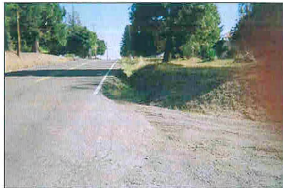
Mountainview will require widening to accommodate bicycles, pedestrians, and motor vehicles safely.
