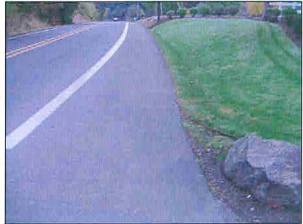
The wide shoulder can easily be striped with a bike lane stencil with the appropriate signage to prevent on-street parking.
