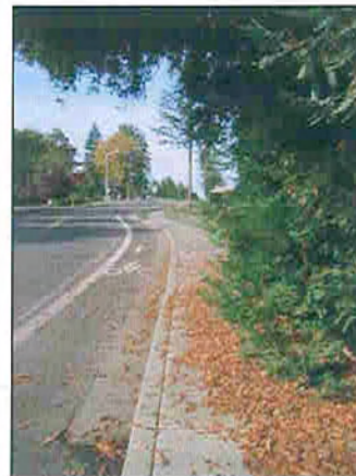
Maintaining existing facilities improves accessibility for all users
