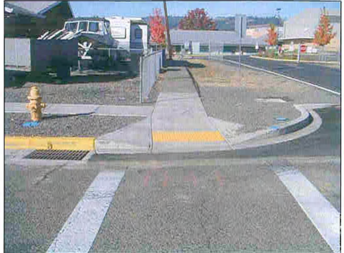
Sidewalk with new curb ramp near high school.
