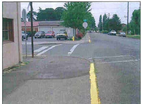
Blaine Street has sufficient roadway width to stripe bike lanes with the removal of on-street parking.
