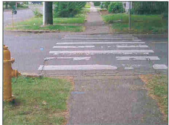
Most of the intersections along River Street are lacking curb cuts, making pedestrian travel difficult for all users.
