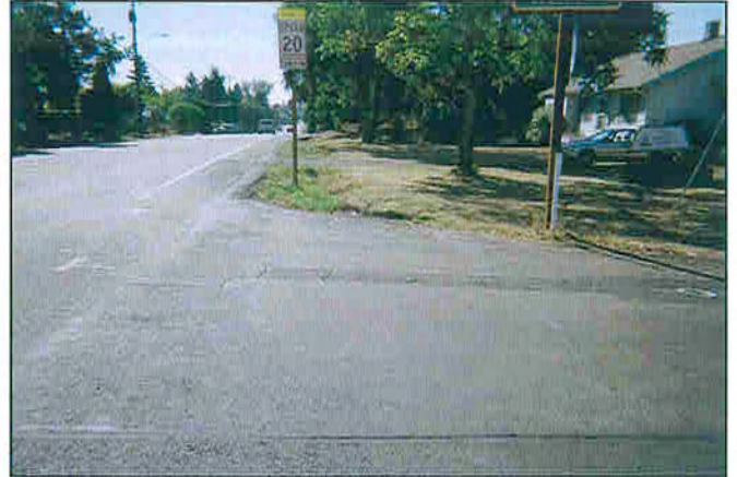
The drainage ditch will have to be piped to accommodate any roadway widening project designed to add sidewalks and bike lanes to College Street.
