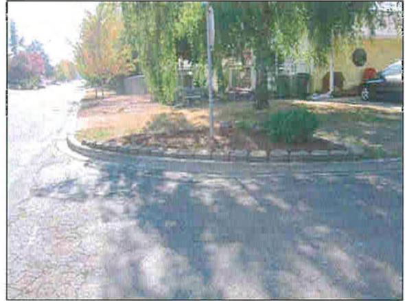
The lack of sidewalks forces pedestrians into the street and competing with vehicle traffic.
