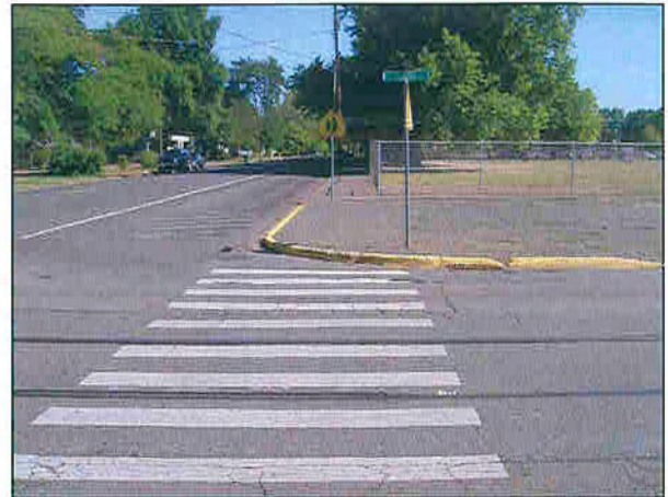
The lack of curb cuts and sidewalk make it difficult to access the school grounds from Blaine Street.
