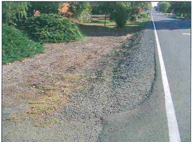
Elliott Road will need to be widened to accommodate sidewalks and bike lanes to meet the functional classification standards.
