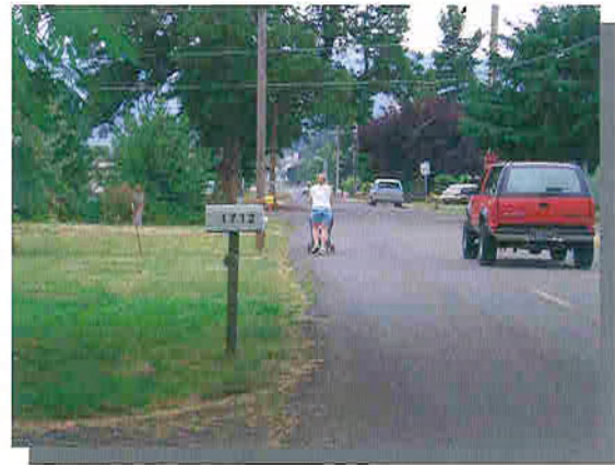
Missing sidewalks force pedestrians into the road, decreasing safety for the pedestrian.
