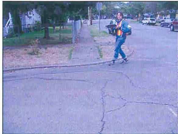
Wynooski has sidewalks close to downtown, however the lack of curb cuts reduces accessibility for all users.
