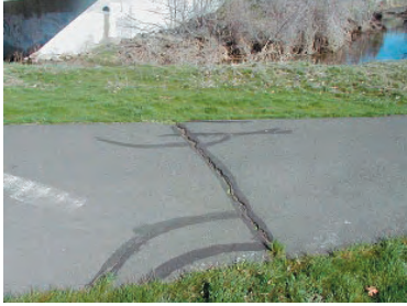
Existing cracks in Willow Creek Trail
