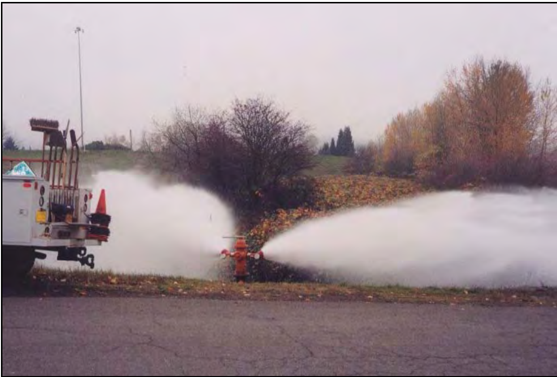
Figure 5-1. Agnes Avenue Hydrant Flow Test
