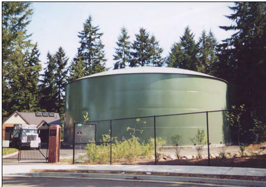
Figure 2-15. Barlow Crest Reservoir
