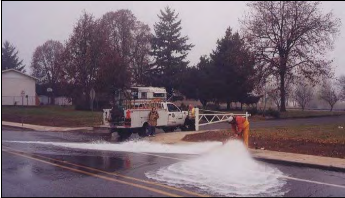
Figure 5-5. Hydrant Flow Test at Clairmont Way
