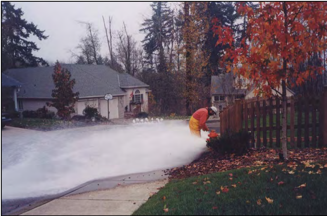
Figure 5-3. Hydrant Flow Test at Gilman Drive
