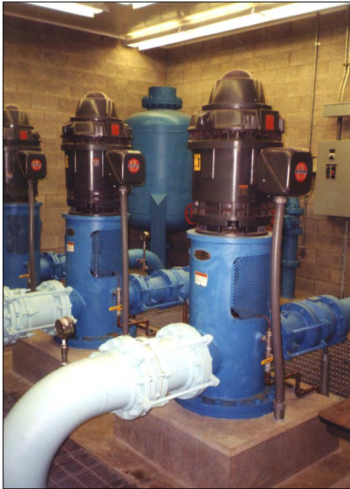
Figure 2-9. Hunter Avenue Pump Station
