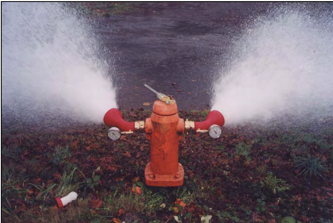
Figure 5-2. Flowing Hydrant at Spring Street
