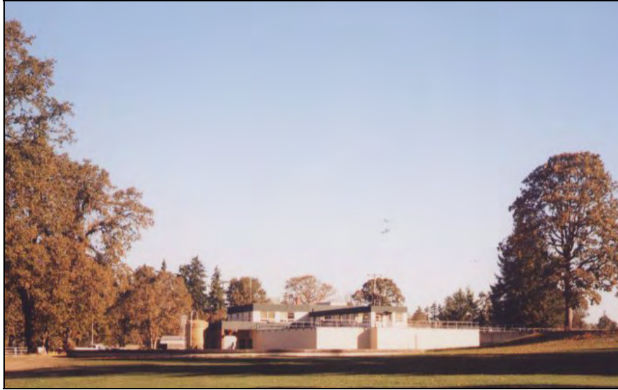
Figure 2-17. SFWB Water Treatment Plant
