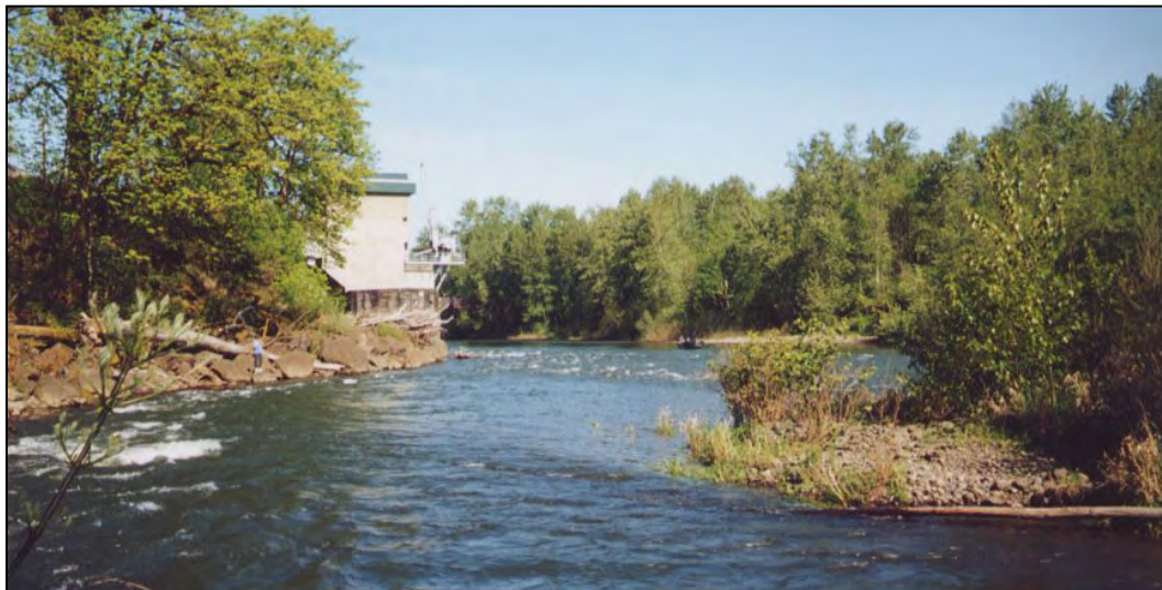
Figure 2-1. South Fork Water Board Raw Water Intake
