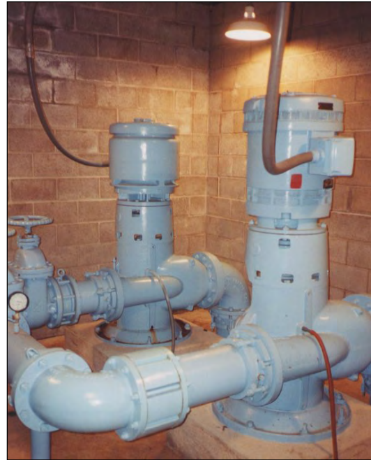
Figure 2-10. Boynton Pump Station
