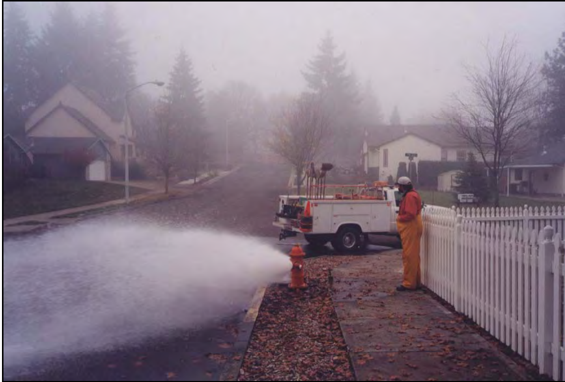
Figure 5-4. Hydrant Flow Test at Clearbrook Drive
