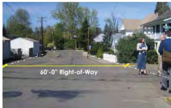
Existing Douglas Street (Railway to Spruce St)
