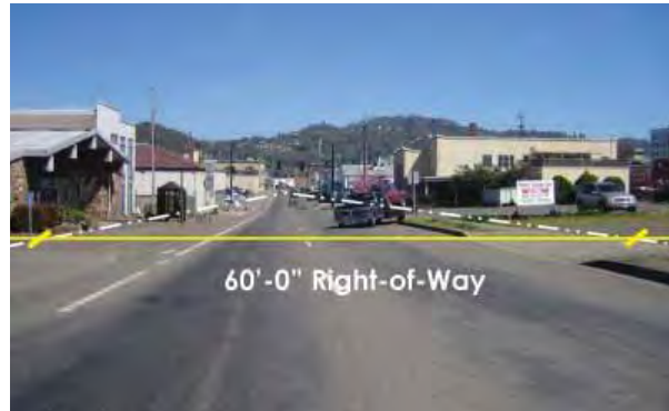
Existing Pine Street (Oak St. to Mosher St.)
