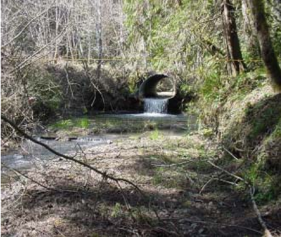
Photo 1 – Culvert on lower Lee Creek
