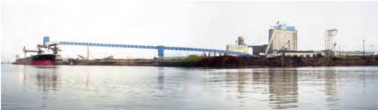
In contrast to a seawall riverbank, the long-arm design of the ship-loading facilities at some marine terminals, such as this bulk terminal at Port of Portland Terminal 4, allows most of the riverbank to remain relatively undisturbed. This is an example of how site design can meet both industrial and natural resource objectives.
