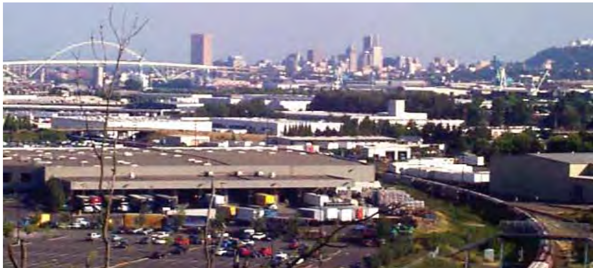
Central location and solid truck, rail, and harbor access are among the locational advantages of the Swan Island industrial district (shown here) for manufacturing and distribution firms.
