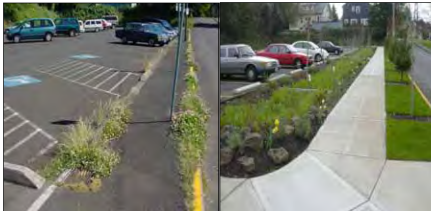
Figure 2-2: Retrofitted parking lot. Before and after pictures show how this parking lot was redesigned to allow rain to soak back into the ground instead of entering the local sewer system.
