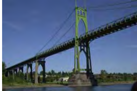
St Johns Bridge
