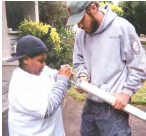
Community volunteers work to disconnect a residential downspout.
