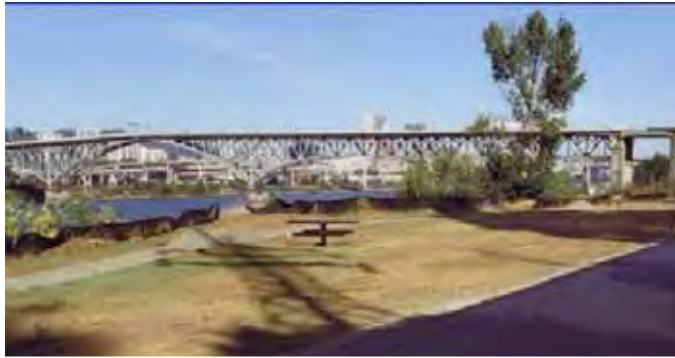
Newly constructed riverfront trail connecting the Central Eastside to the Springwater Corridor Trail. It is approximately 14 feet wide.
