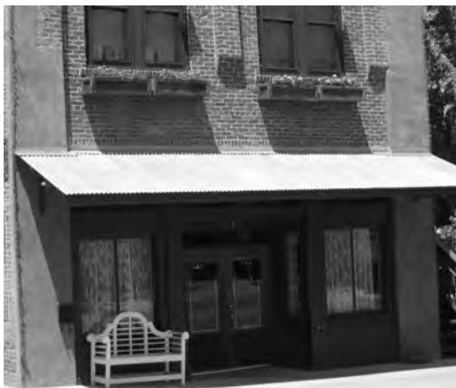
Figure 36: An open-sided corrugated metal awning
