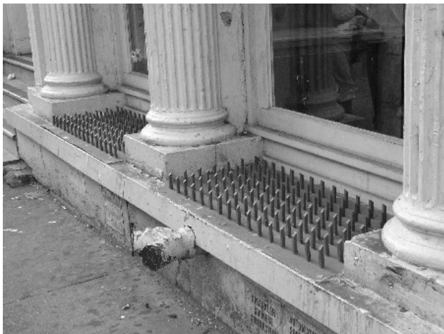
Figure 39: Anti-Sit devices includes spikes or other elements that discourage pedestrians
