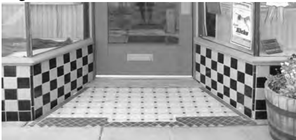
Figure 27: Surface treatment in recessed entries defines private v. public right of way, creating a sense of entry.
