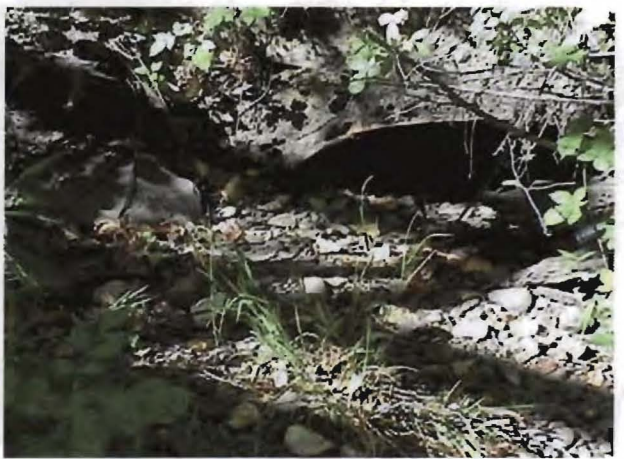
Photo 6. Culvert at Allen Street filled with sediment.
