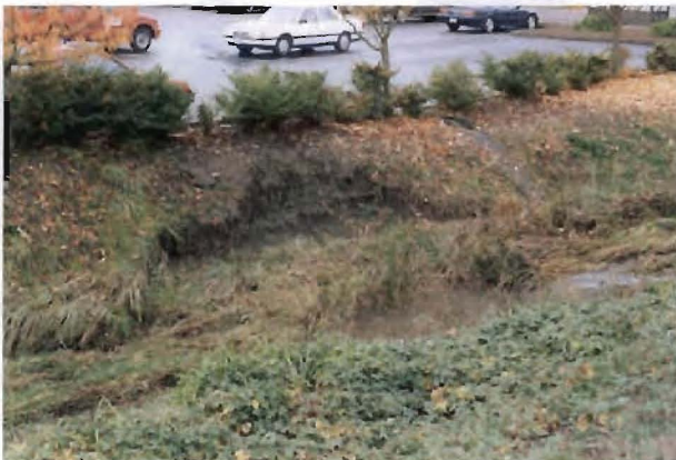
Photo 5. Parking lot runoff at Avery Square Shopping Center
