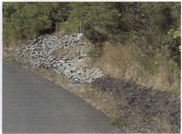
Photo 6. Park Estates ditch with riprap
