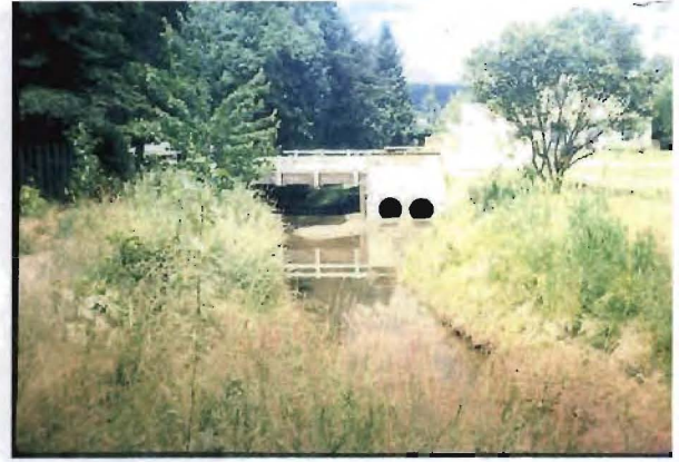
Photo 4. New culverts at Garfield Avenue
