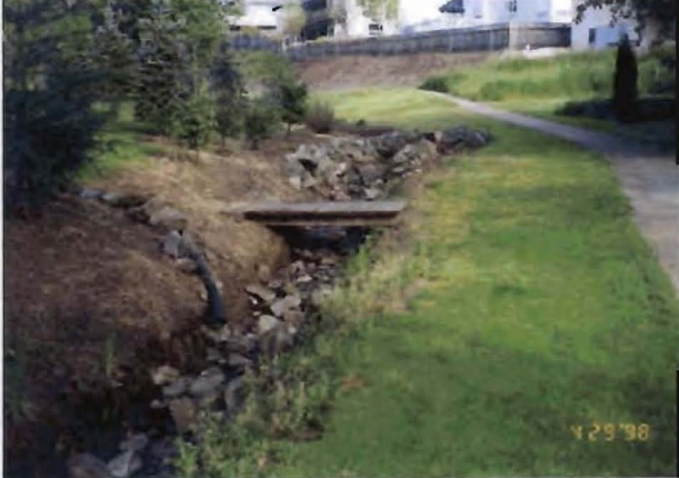
Photo 6. Upstream landscaping near Chipmunk Place
