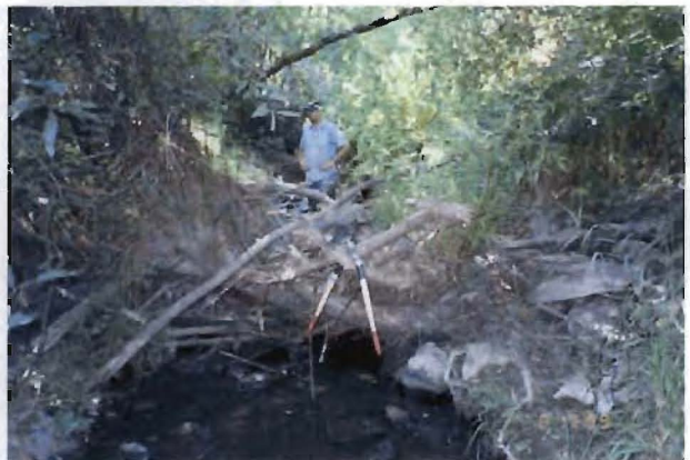
Photo 6. Stream blockage downstream of Knollbrook Place
