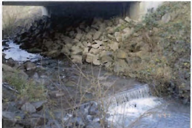
Photo 4. Fish passage concern at Brooklane Drive
