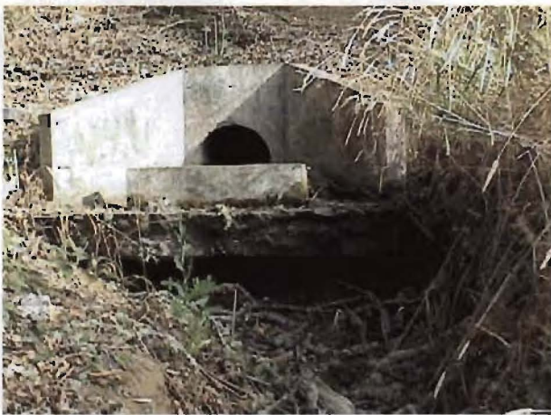
Photo 5. Erosion at east culvert outlet
