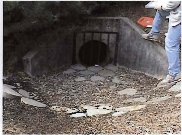
Photo 4. Entrance to east culvert in private yard
