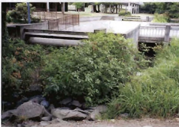
Photo 5. Jackson Creek at courtyard area at CVHS
