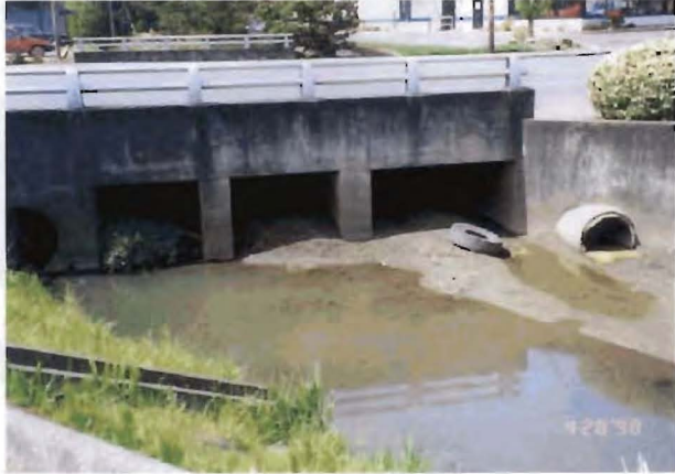
Photo 5. Culverts at Ninth Street
