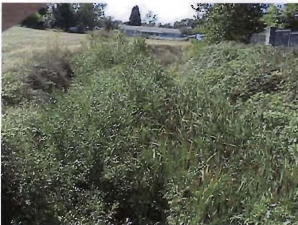
Photo 3. Channel upstream of Crystal Lake Drive.
