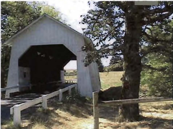
Photo 5. Irish Bend Bridge along Campus Way
