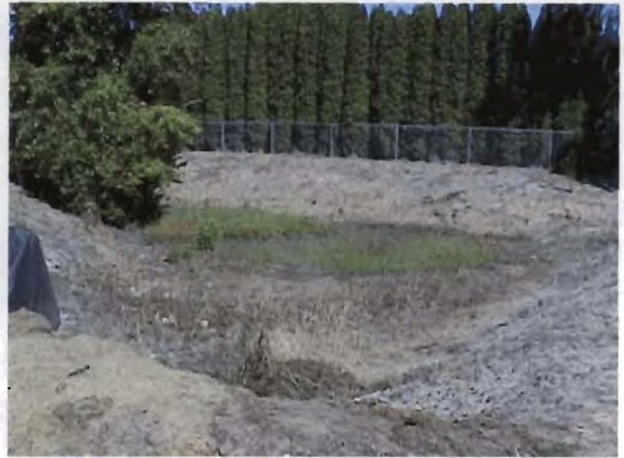
Photo 2. Detention pond near Goodnight Avenue.
