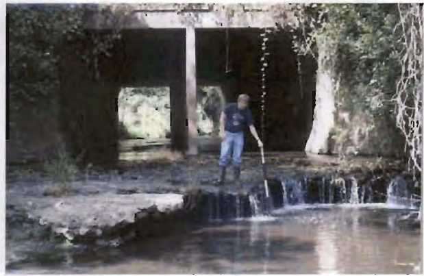
Photo 2. Fish barrier at Hwy 20/34
