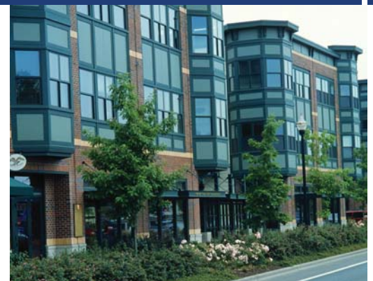
View of the Orenco Station development
