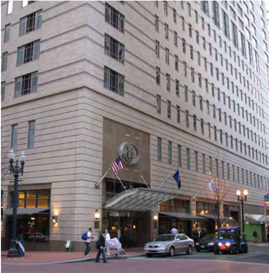
The sloping floors of the parking garage for the Hilton Expansion are masked with the building facade's use of regularly spaced windows that mimic the hotel windows of the floors above.
