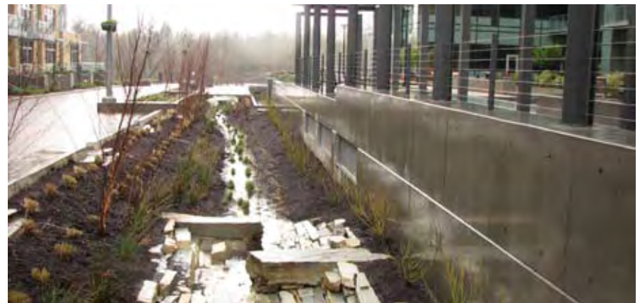
Both the Meriwether (top) and Atwater Place (bottom) include stormwater catchment areas along Pennoyer Street. The design of the landscape allows the areas to serve as both a water feature, landscaped buffer, and critical stormwater function that is attractive with or without water.
