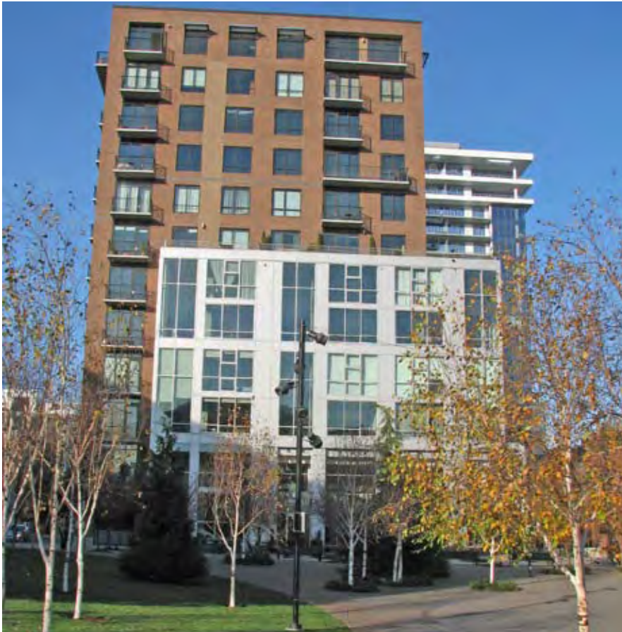
The massing of Park Place Condominiums steps away from Jamison Square, allowing light and air to filter into the open space.
