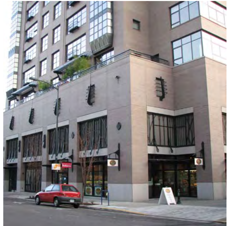
Retail and facade ornamentation on the lower levels of the Elizabeth mask a parking structure, effectively screening views of parked cars and providing an active street environment for the pedestrian.
