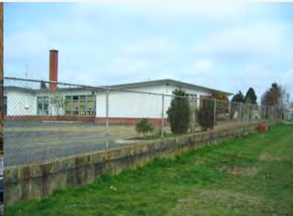
School/community border at Faubion
