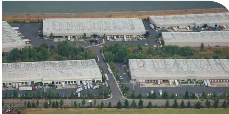
Columbia corridor warehouses
