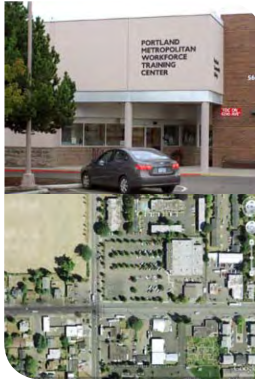
Portland Metropolitan Workforce Training Center - aerial
