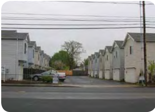
The design overlay zone is less frequently applied to development in lower density multi-dwelling zones such as this development in the R3 zone.
