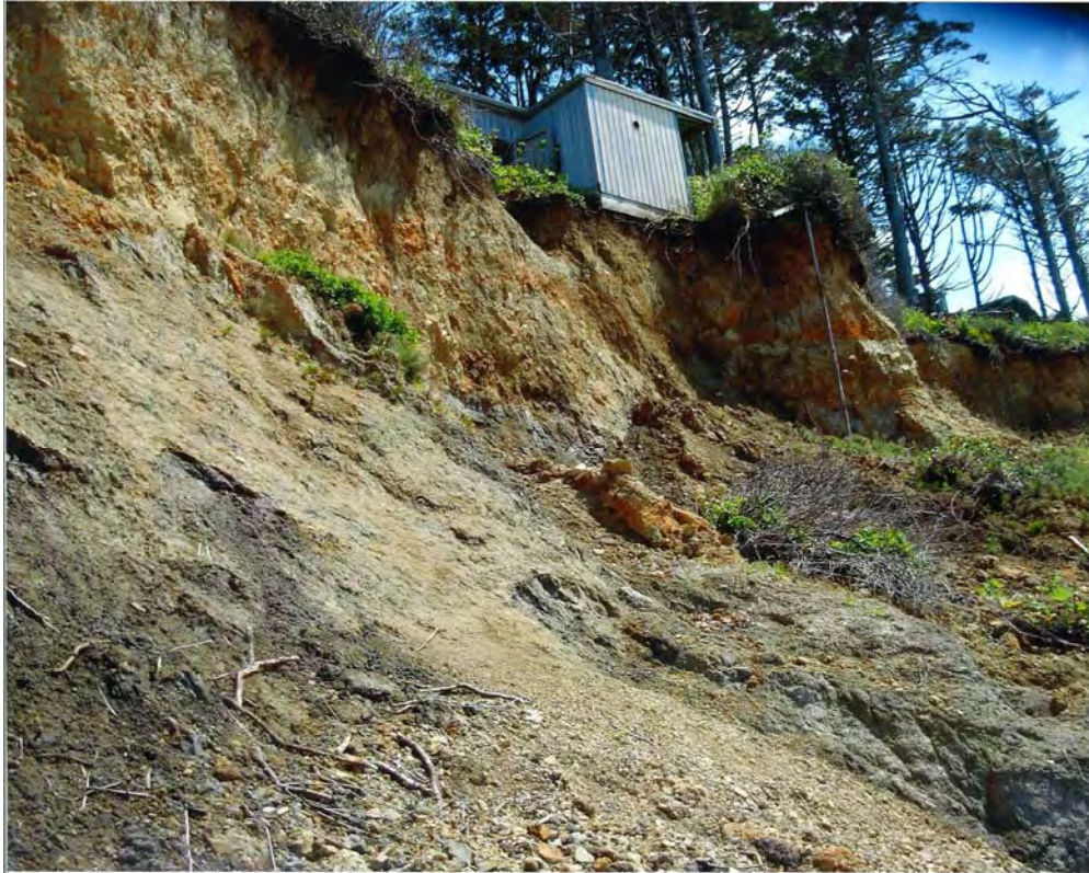
An example of coastal erosion near Arch Cape. (2008 Clatsop County photo)
