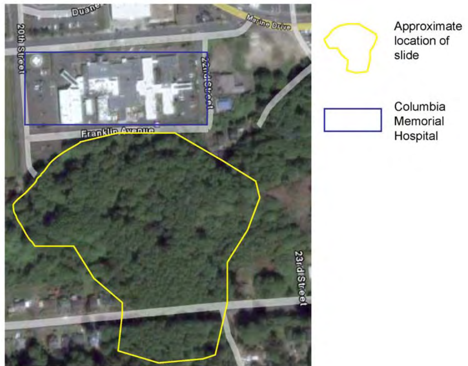
Figure 13. Historic Landslide Impact Area – Astoria, Oregon
