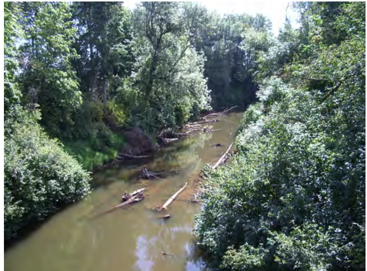
Site 15: Bridge crossing at the Luckiamute River (Station 260+00).
