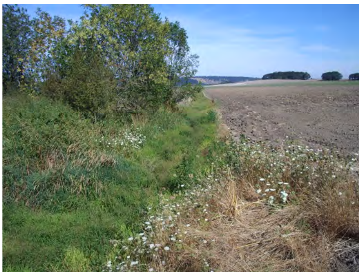
Site 5: Drainage ditch near NW Ryals Avenue (Station 135+00).
