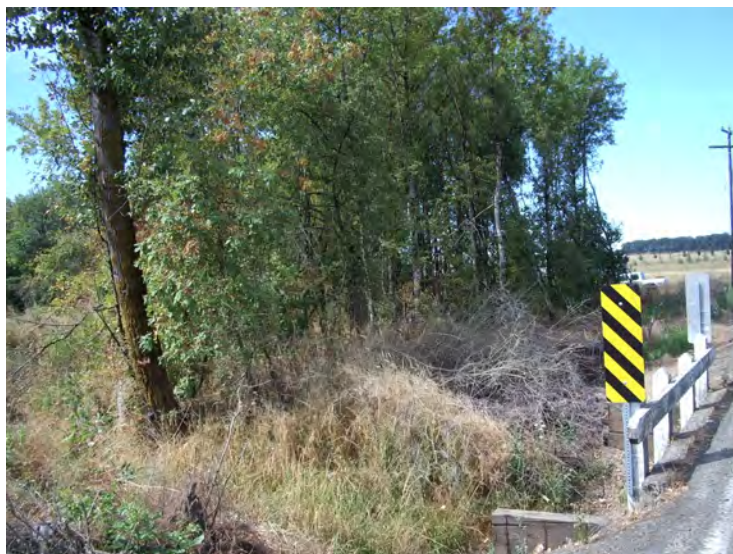
Site 22: Unnamed creek crossing near Stapleton Road (Station (605+00)).
