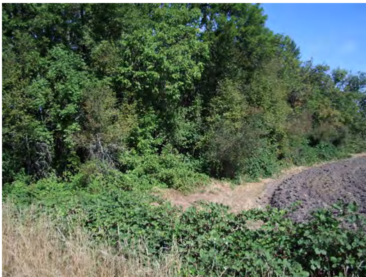
Site 8: Forested wetland at culvert crossing on Camp Adair Road (Station 20+00).
