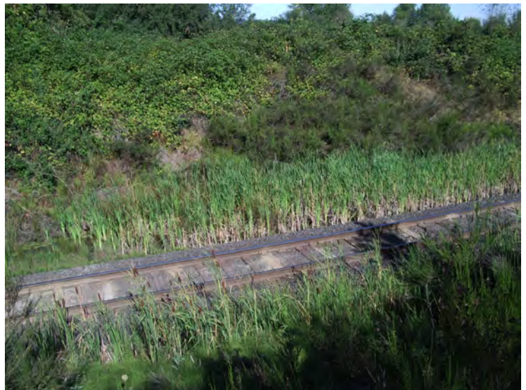
Site 7: Large drainage at SP Railroad crossing (Station 100+00).
