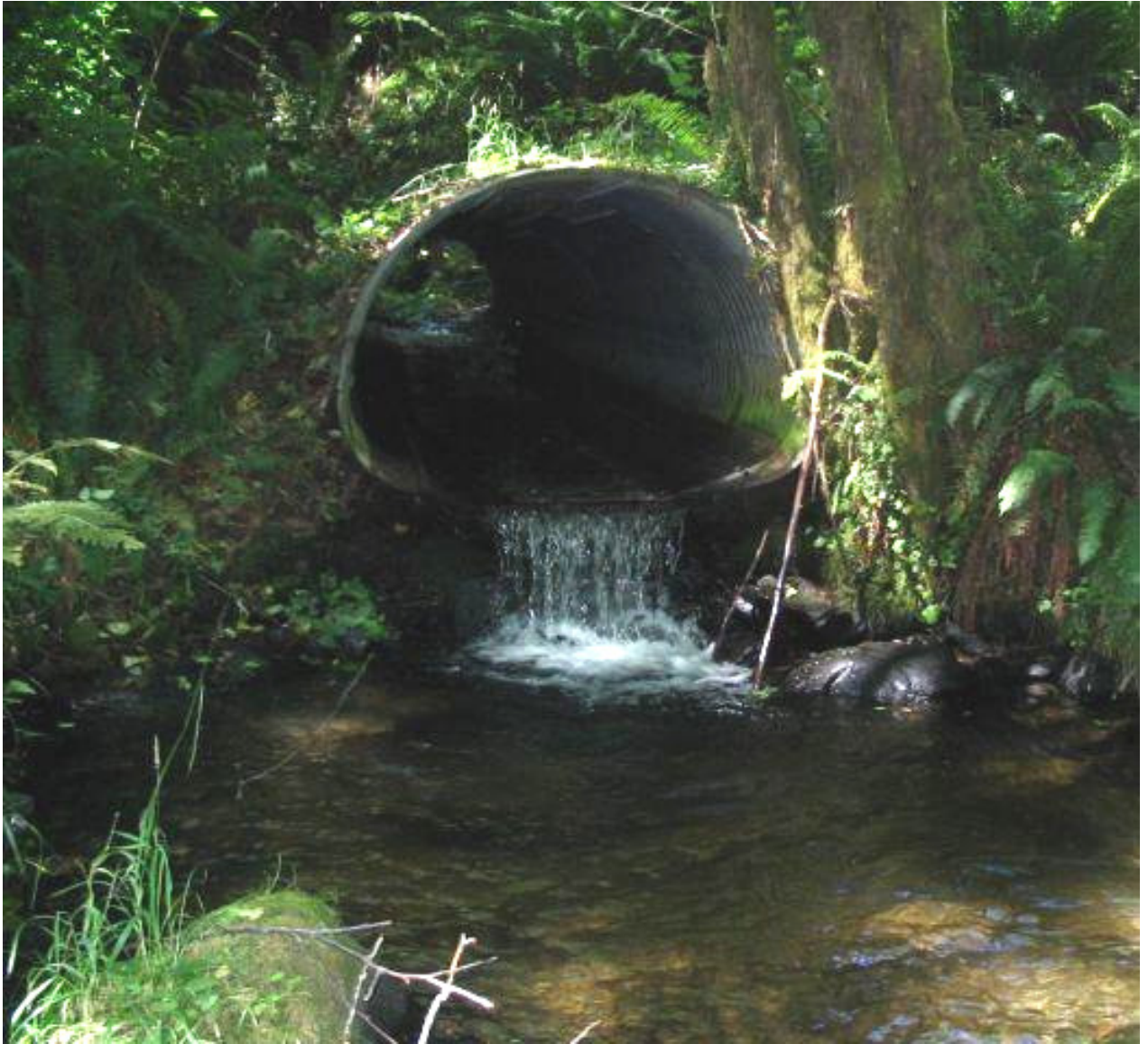
Culvert blocking Fish Passage on West Fork Mill Creek in the Lower Alsea River Watershed (2008).
