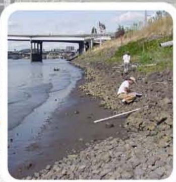
Morrison Bridge East: A steep, rock-armored bank is constrained by a narrow river channel and trail/freeway development at the top of bank. Scattered non-native vegetation exists on the bank.
