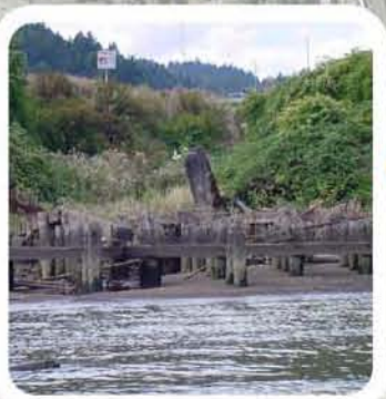
Zidell Ross Island Bridge: The inactive industrial site riverbank has rock rip rap and construction debris, and remnants of a pile-supported dock. Sparse bank vegetation is dominated by non-native blackberry.
