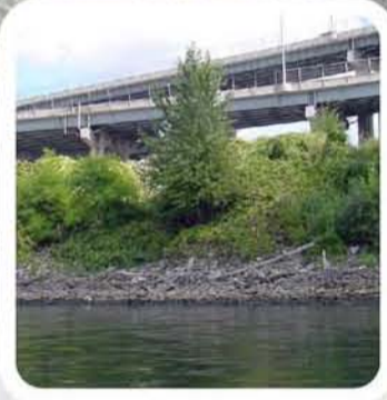
Eastbank Crescent: This is a fairly steep, rip rap covered bank with non-native blackberry as the dominant vegetation. The near-shore area is shallower nearest to the Hawthorne Bridge.
