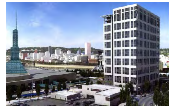
Block 49 - 19 Story Office Building
