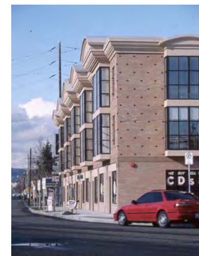
Sidewalk width will be 15 feet from face-of-curb. Bay windows, overhangs and building extensions above the first floor can increase floor area and contribute to the distinct character of the street.
