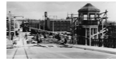
By 1926 the new Burnside Bridge was nearing completion. The draw bridge tender's tower and streetcar system are shown here in the foreground.
