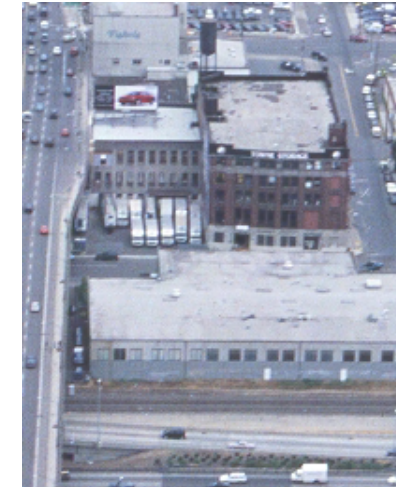
Towne Storage building on the upper right.
