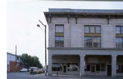
Burnside is lined with a variety of historic and contemporary buildings. Many older buildings have detailed brick work and attractive architectural features but are in poor repair.
