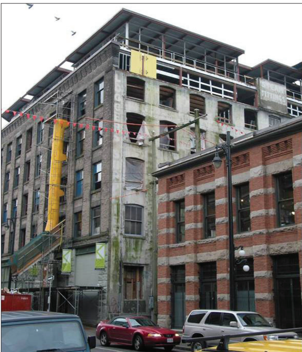
New construction adjacent to old in Gastown.
