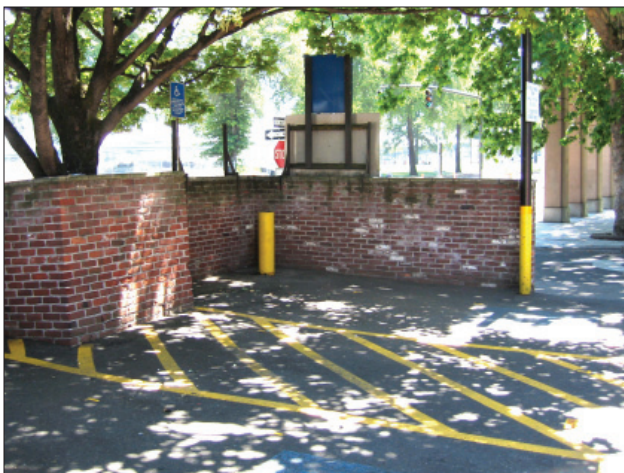
Parking entries such as this, fronting upon a major event street (Ankeny), should be discouraged.
