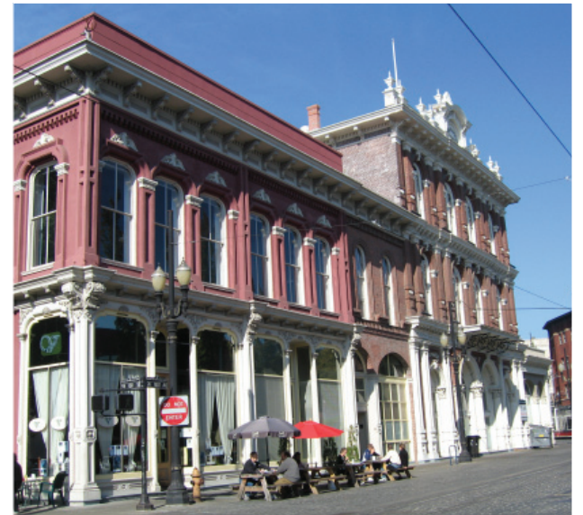
The ground floor is typically taller than the second and higher floors of the District’s historic buildings.
