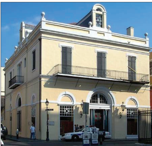
Vieux Carre architecture.
