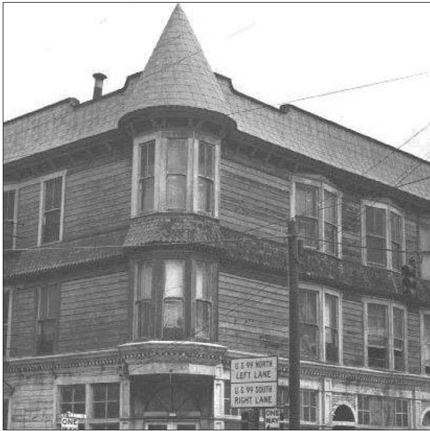
Wood-frame building at 3rd and Morrison, construction date unknown. Photo date 1961. Early commercial buildings downtown were wood frame, later replaced with more “fire proof” brick.
