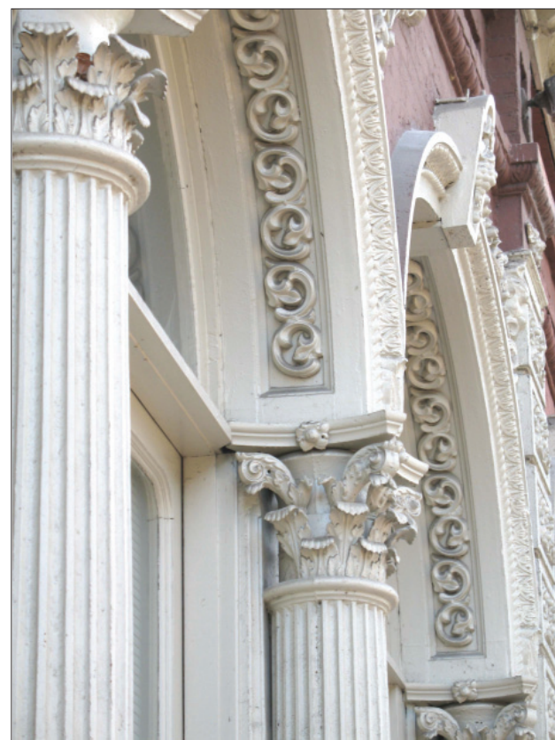
The reuse of cast iron should be encouraged, where appropriate.
