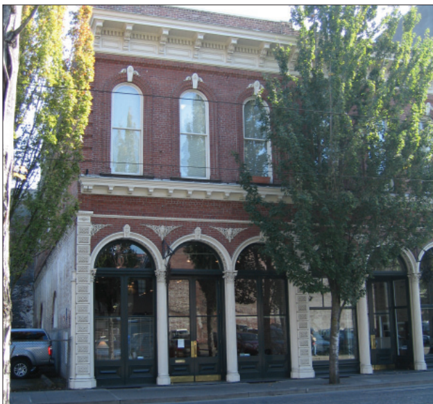
Cast iron is a prominent feature in many of District historic structures.
