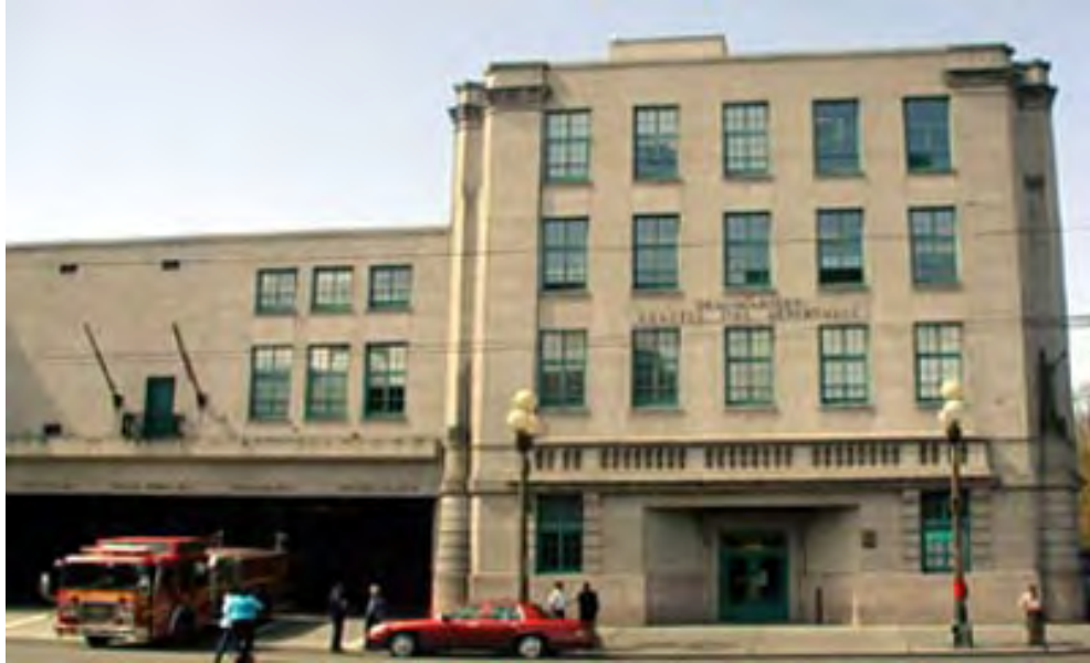
Fire Station 10, Pioneer Square, Seattle, WA
