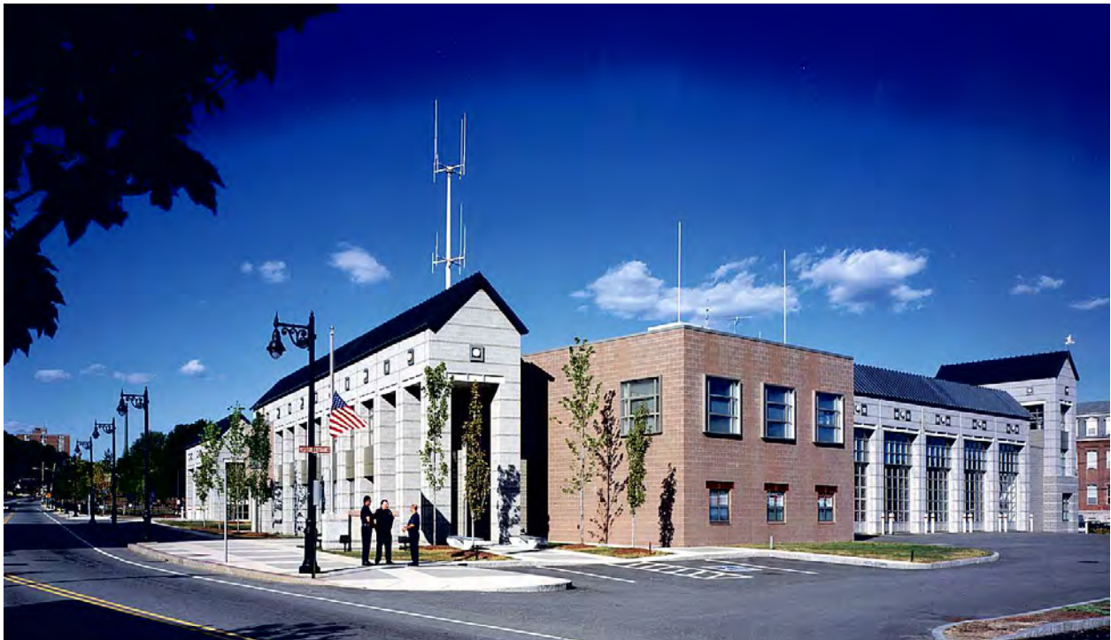
Central Fire Headquarters, Fitchburg, MA
