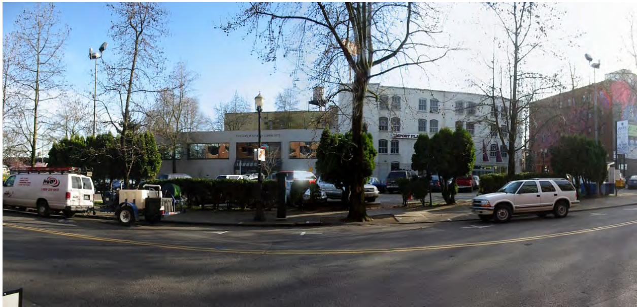
Block 8, as viewed from the north
