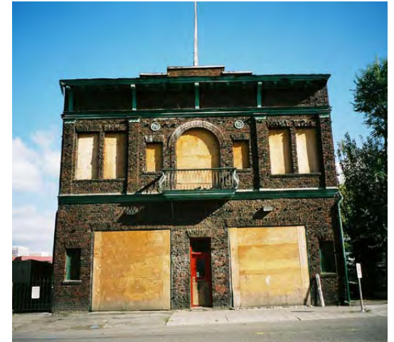
Engine House #2, Block A&N
