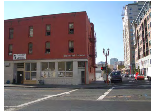
The Blanchet House of Hospitality structure, looking south from Glisan Street and Fourth Avenue
