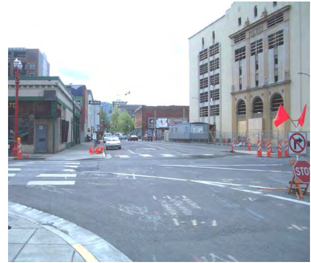
The existing asphalt expanse on Glisan Street, between 3rd and 4th Avenues, as seen from the east
