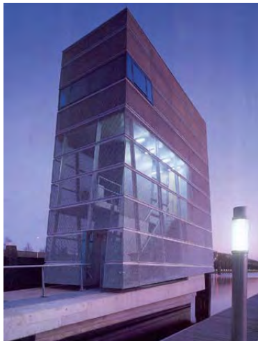
Wire Mesh Cladding Bridge Control Office, Netherlands
