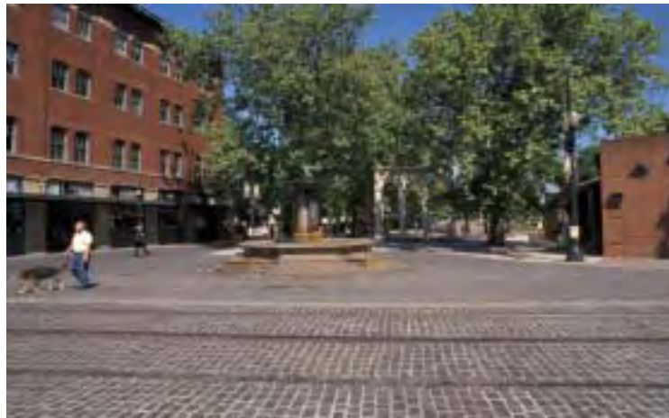
ANKENY PLAZA is one of Portland's most promising urban spaces, but it is surrounded by parking lots, blank 'art' walls at Fire Station 1 and poorly performing retail. The plaza is empty most days of the week and evenings. Crime is a problem in the area.
