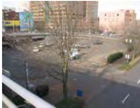
Morrison Bridge Circular Ramp
