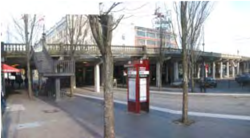
THE AREA BENEATH THE BURNSIDE BRIDGE is a crime area and creates a barrier between the historic district that extends north and south of the bridge, negatively impacting the entire district.
