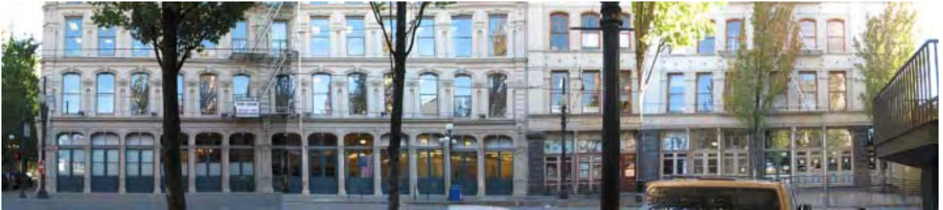
Block 9 on First Avenue
