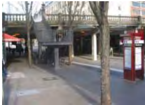
Key Weakness: Public Safety centering on the Burnside Bridge
