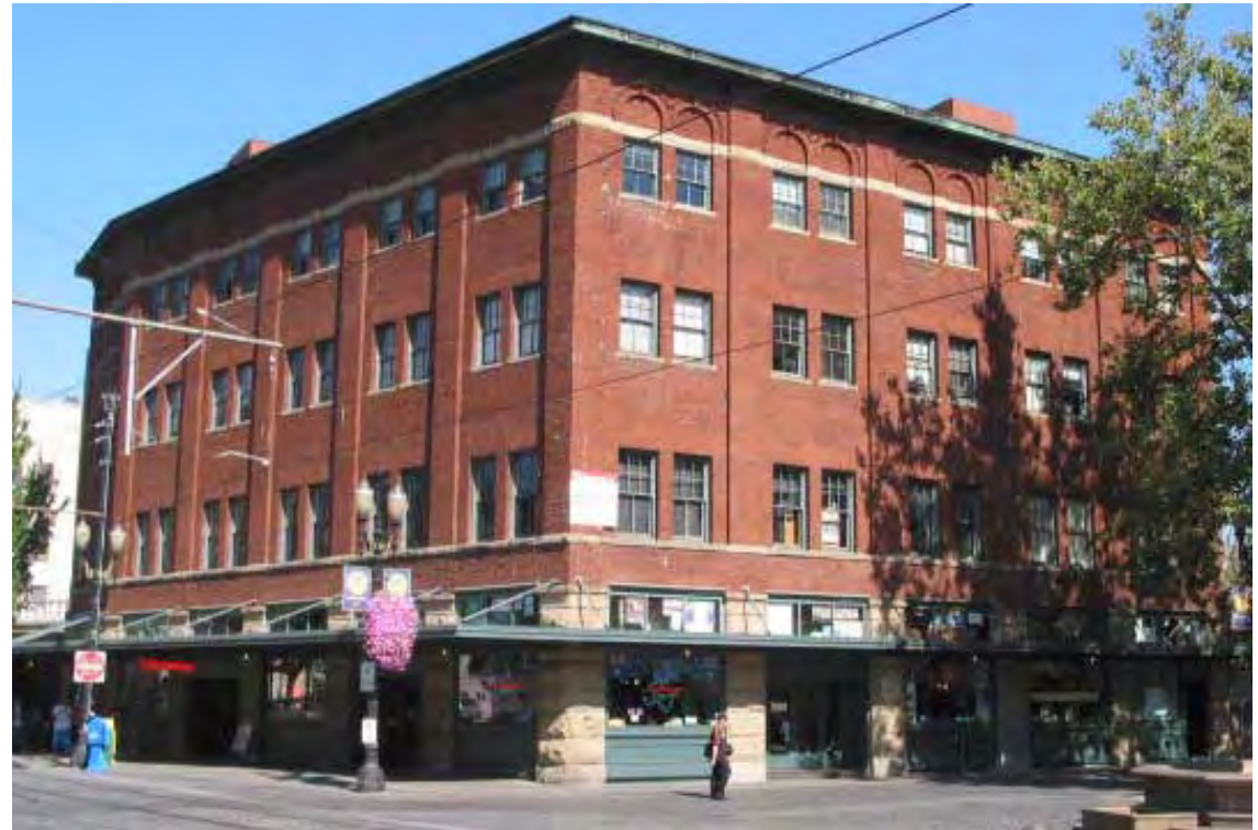
The Skidmore Fountain Building currently.
