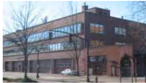
Existing Fire Station 1.
