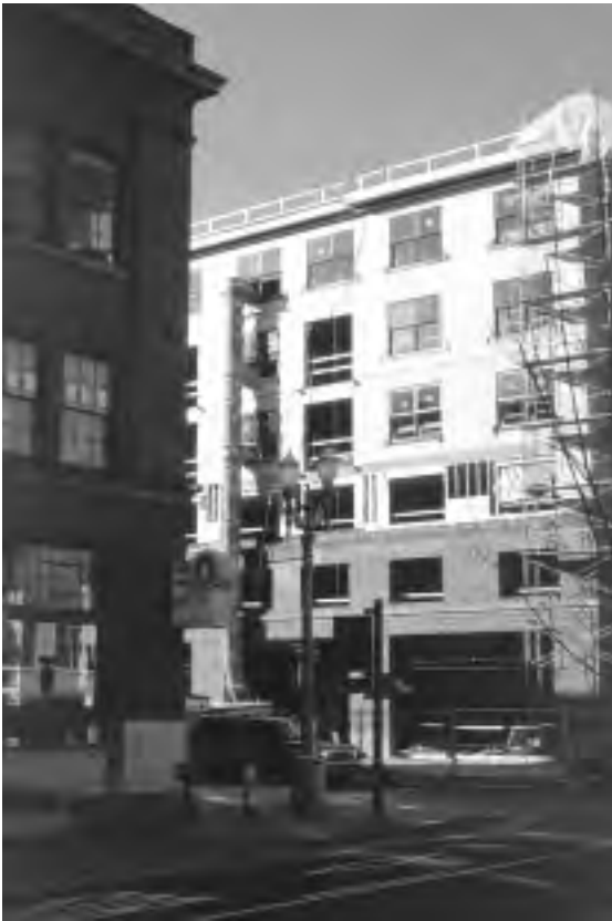
Fifth Avenue Court Apartments under construction
