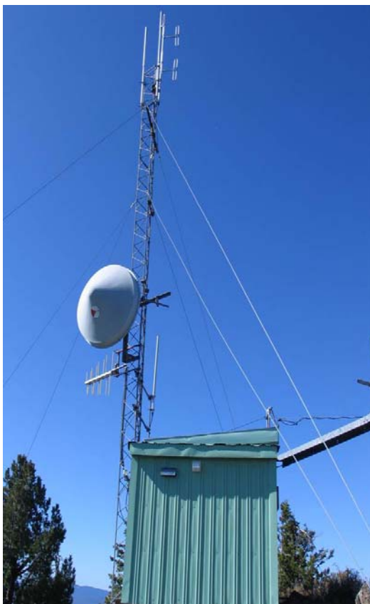
Figure 4. Tower (T1) to be removed from Zone A
