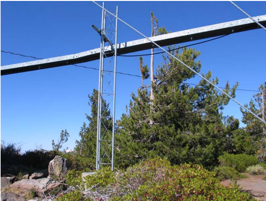
Figure 5. Cable bridge and tower (T2) to be removed from Zone A
