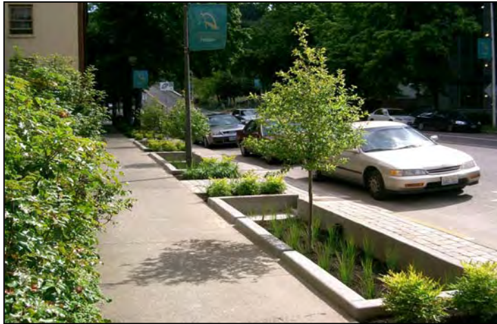
Stormwater planter box with pervious pavers in continuous on-street parking access strip Most appropriate on commercial streets and high density residential streets
