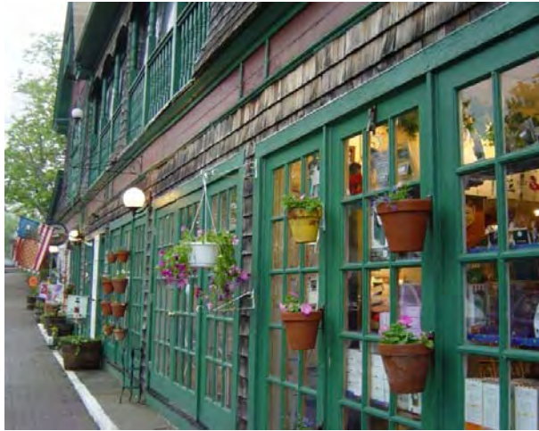
Ground floor multi-pane windows
