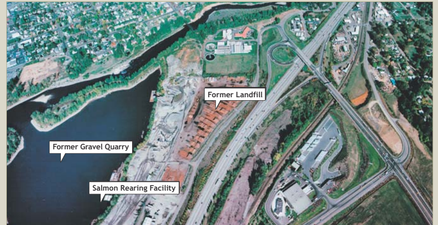
Although most of the industrial activity had ceased by the early 1990s, the impact of these activities is still apparent.
