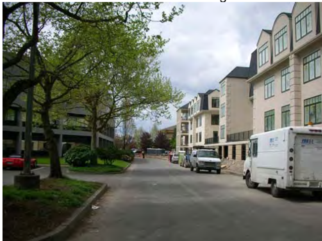
Looking west along north shore of Hayden Island at new multi-story condominium building.
