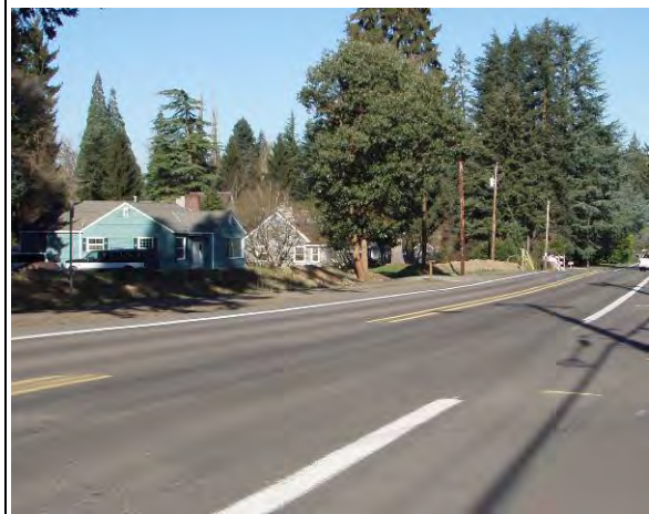
Facing North Upper Boones Ferry Road at Findlay Road
