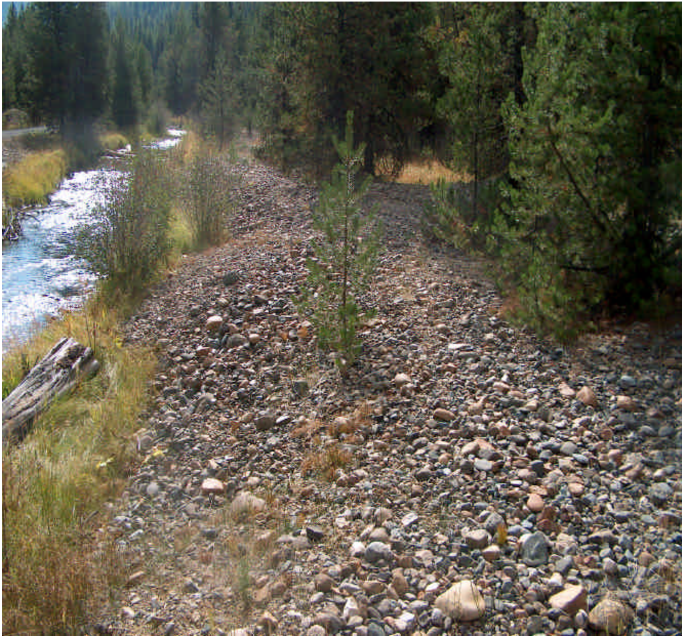
Mine tailings, preventing access to the floodplain.
