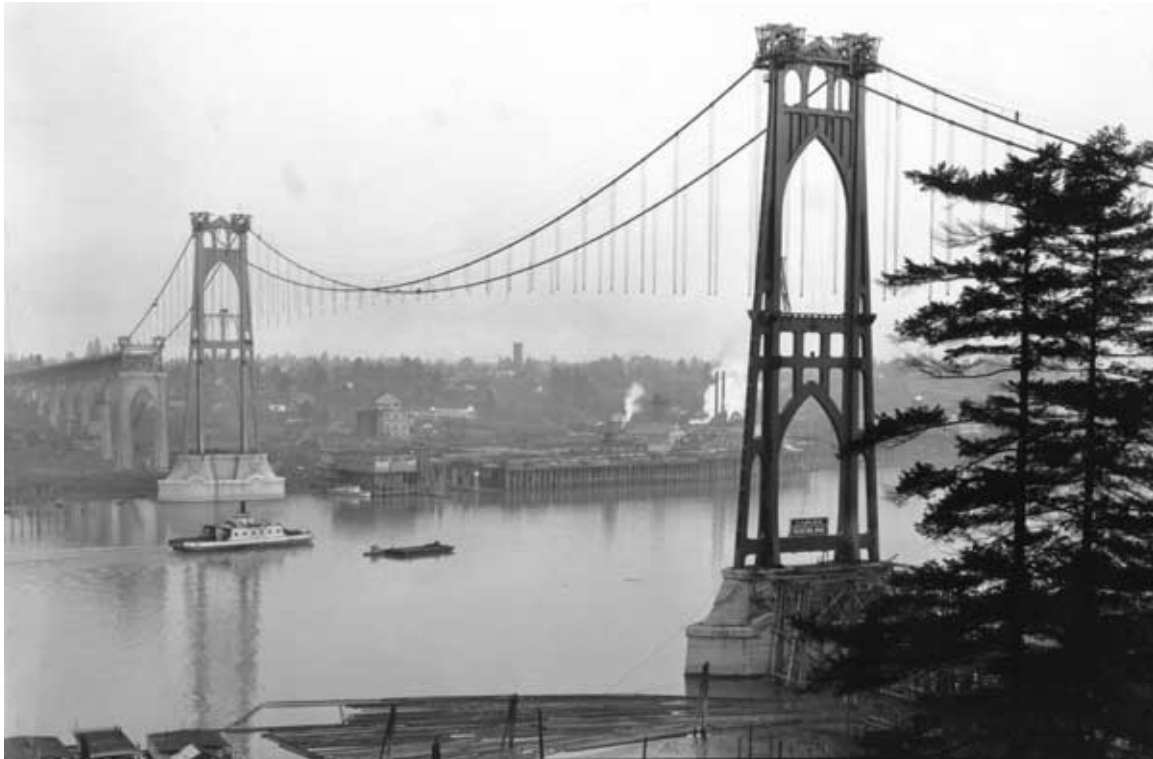
St. Johns Bridge during construction.
