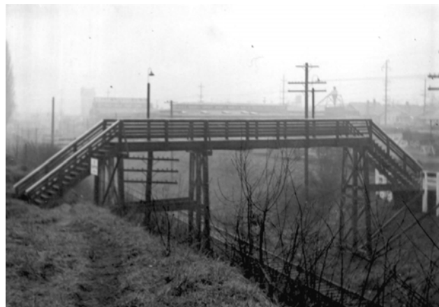
Pedestrian bridge over railroad, Sullivan’s Gulch, near NE 42 nd .
