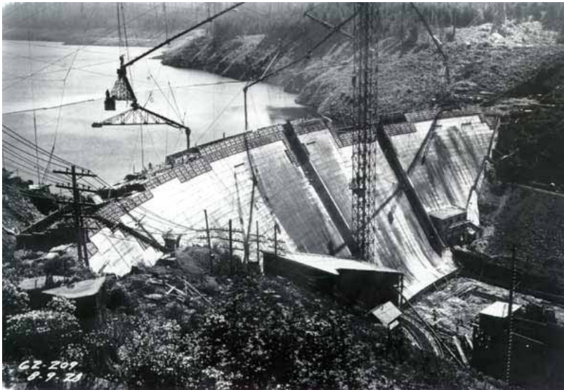
Construction of Bull Run Dam, 1928.
