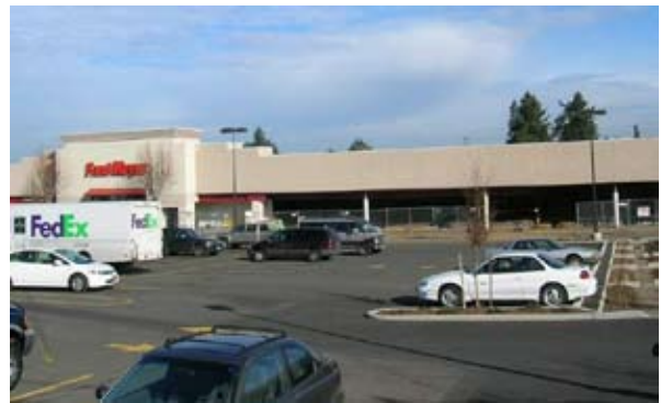
Fred Meyer is undergoing a major renovation and expansion—to be completed in 2007.
