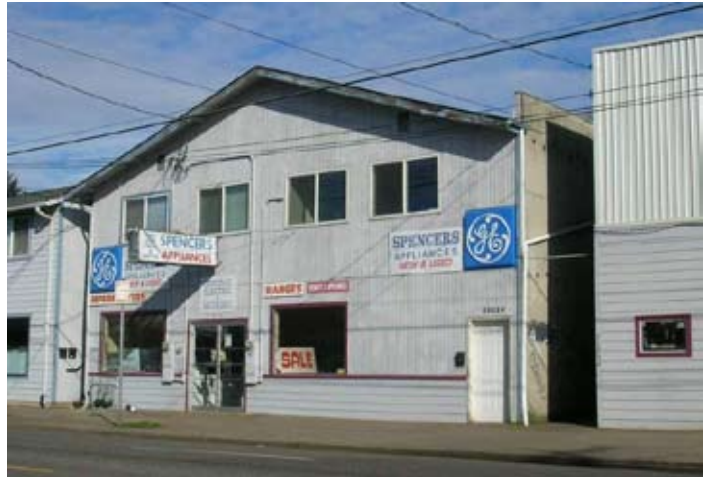
Many storefronts along the corridor show under-capitalized signs and facades which compromises the integrity of the corridor. A sign and façade program would be a useful tool along the corridor.
